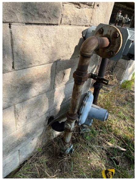
Currently the meter is on the front of the building, and the service line goes through a hole in the sandstone wall. We were unable to access the basement due to safety concerns given the structural integrity of the building.
