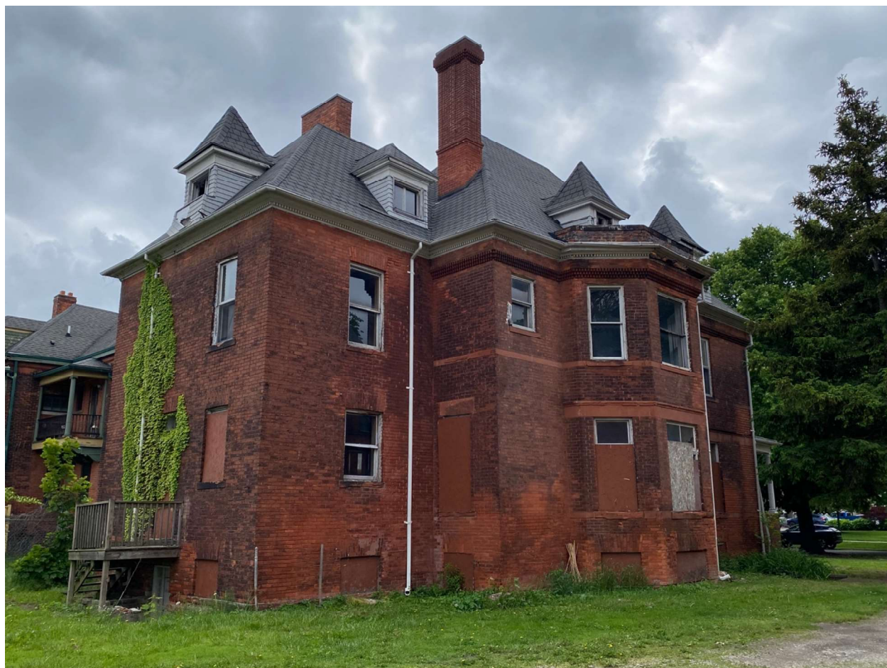
West Side and Rear of House
