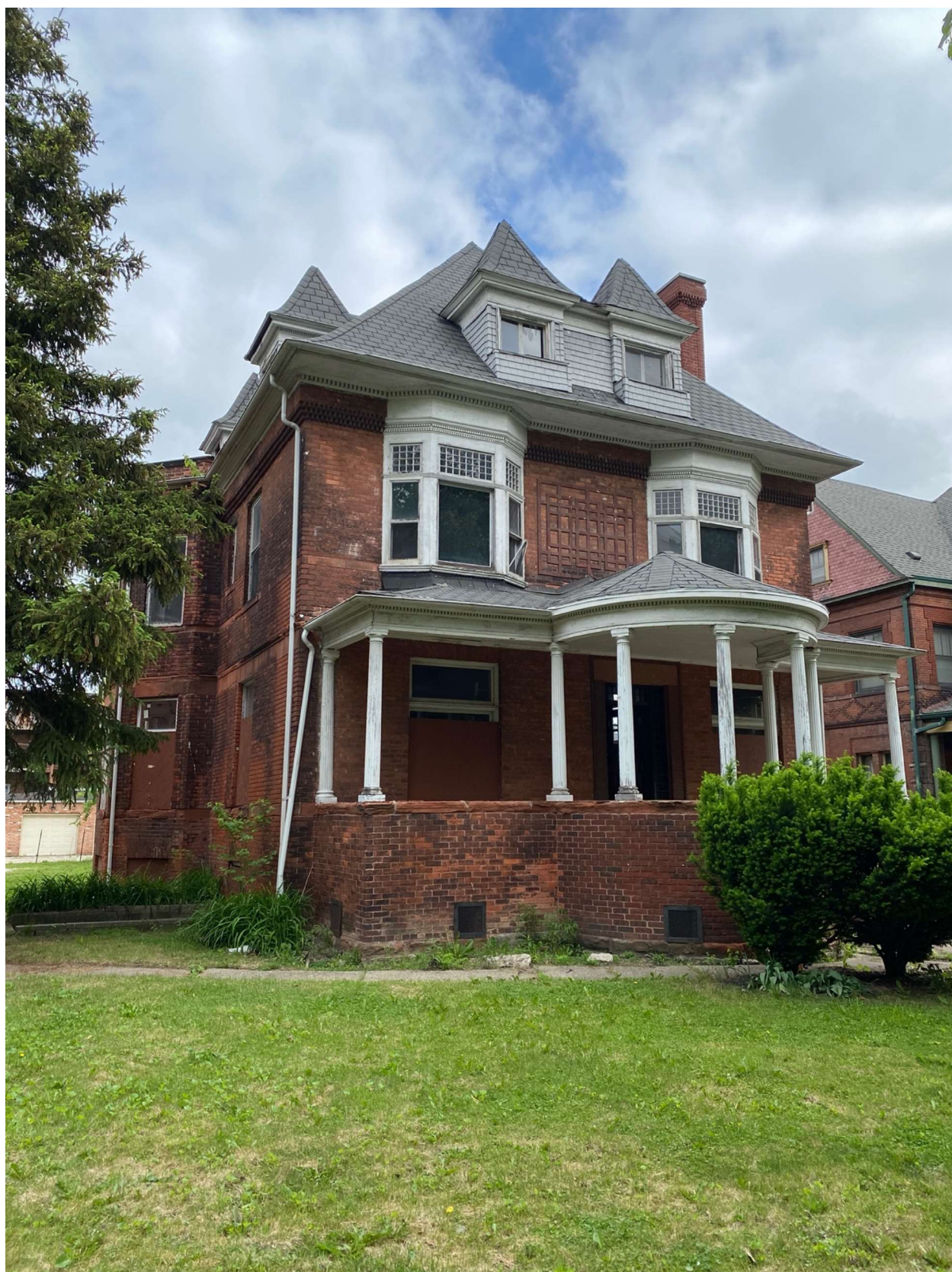
Front and West Side of House
