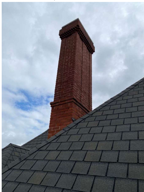
Rear West Chimney
