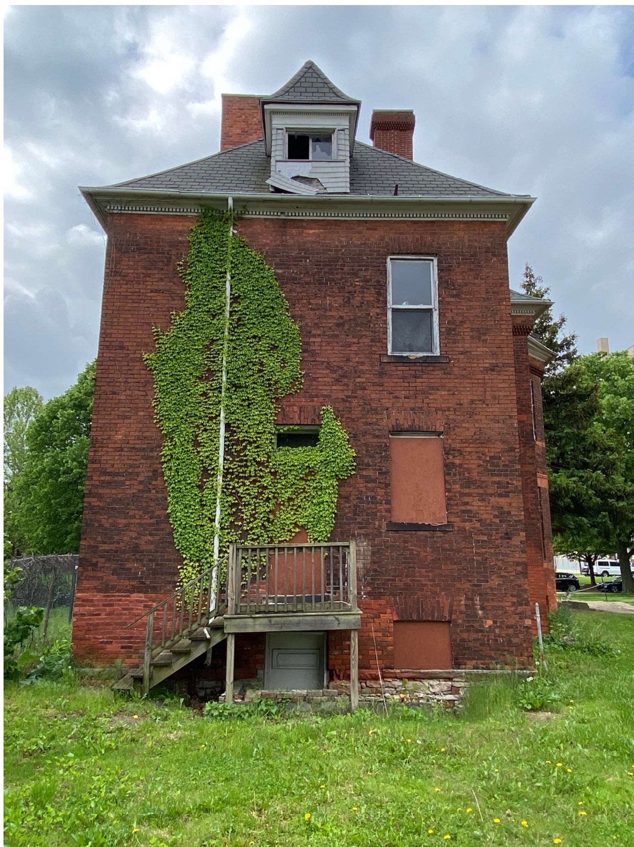
Rear of House
