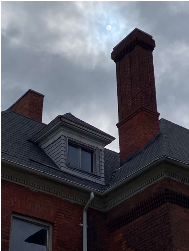
D05 and Rear Chimney
