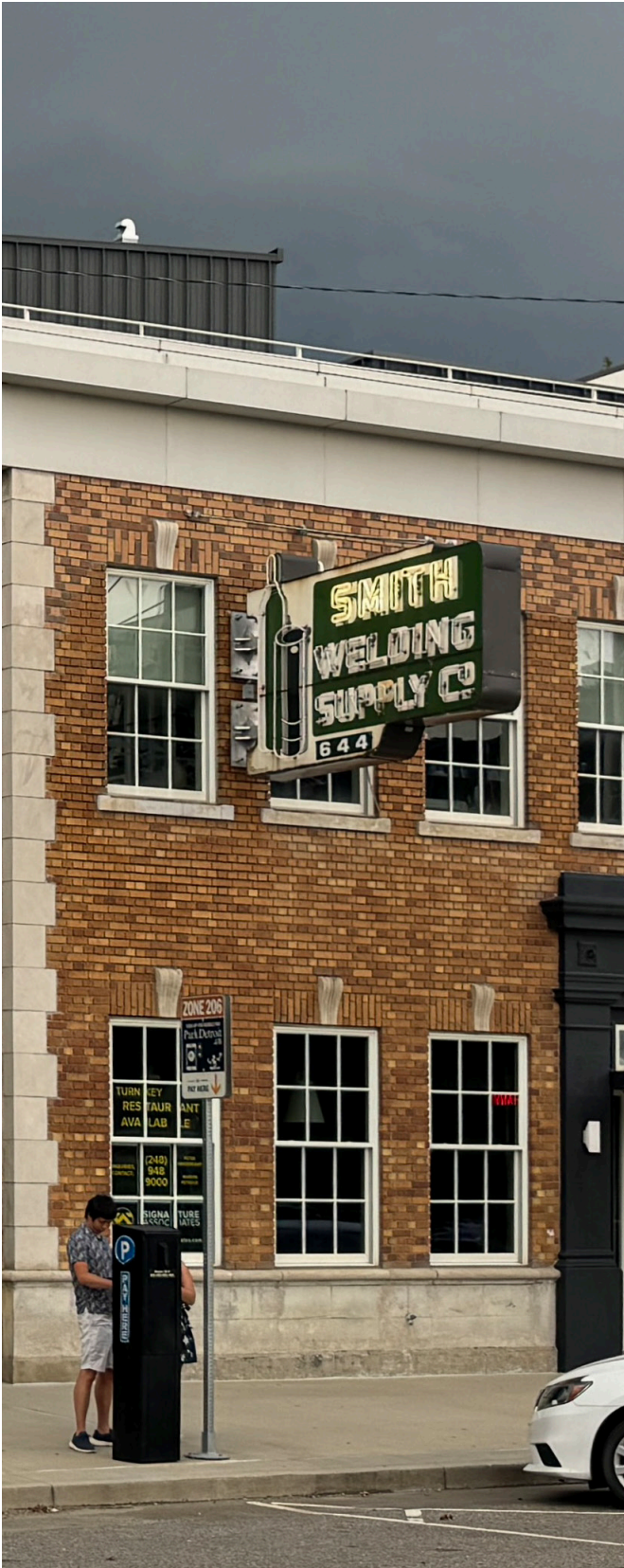
CURRENT ‘SMITH WELDING’ BLADE SIGN LOCATION AT SELDEN STREET
