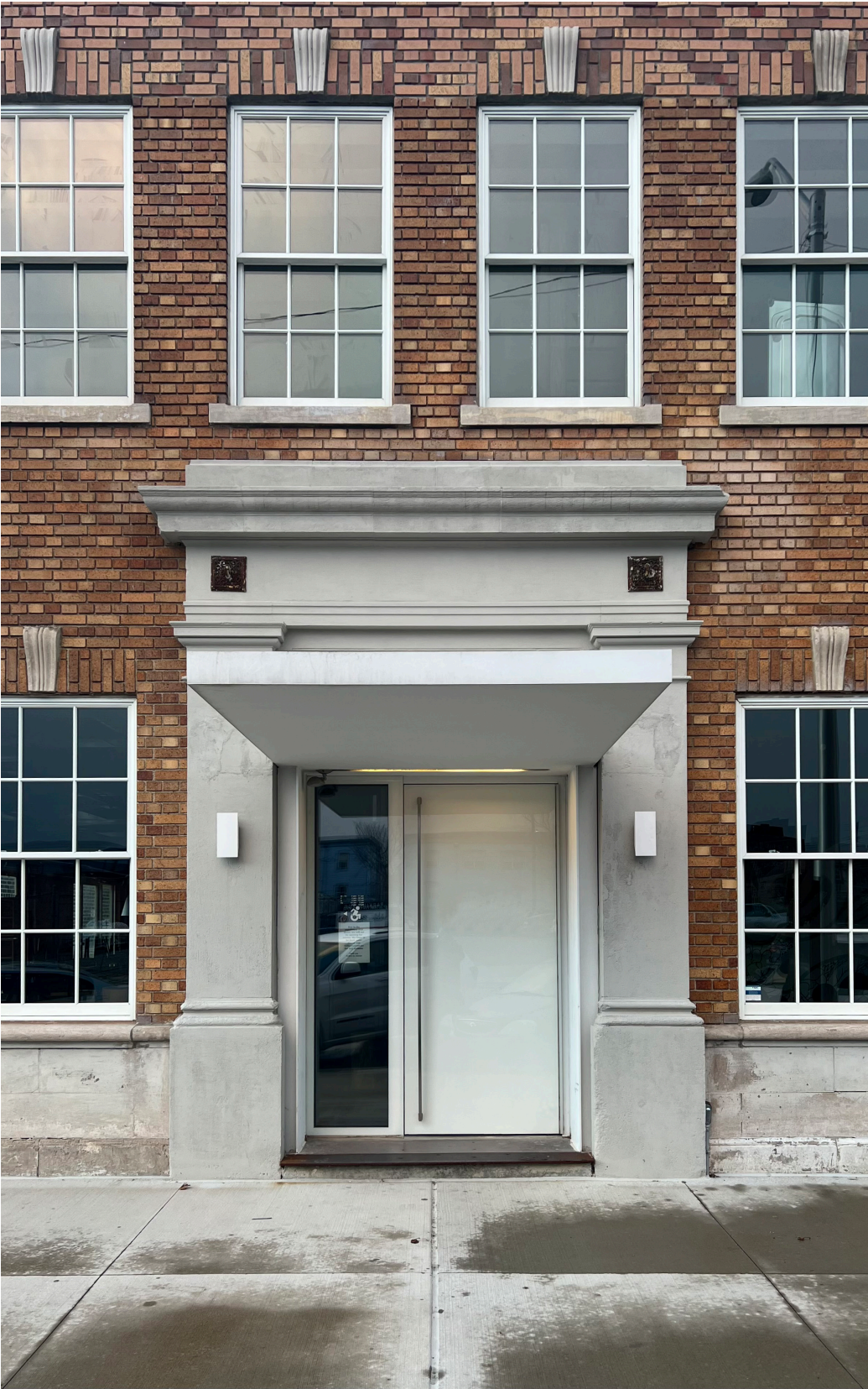
LIMETSTONE PORTAL AND CANOPY, INSTALLED 2019
