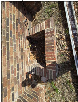
3 SOUTH ELEVATION BASEMENT WINDOW WELL - EXISTING
