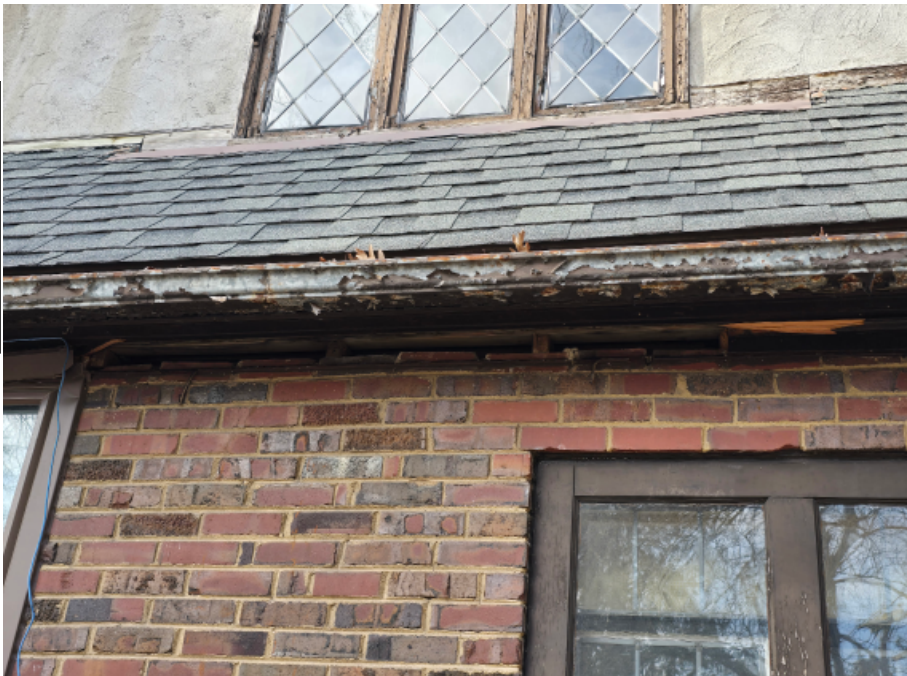
FASCIA/TRIM/GUTTER REPAIRS
