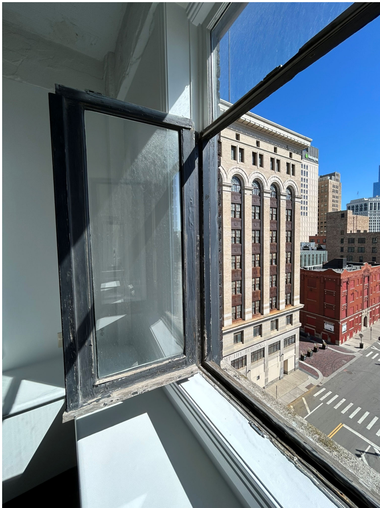
View of existing window sash
