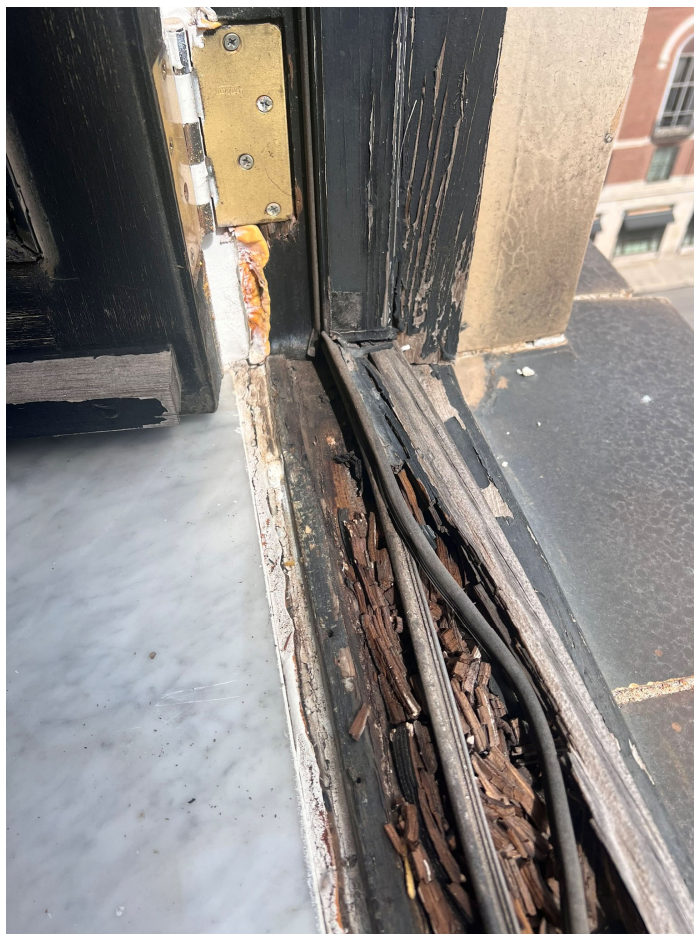
Close up view of window frame sill
