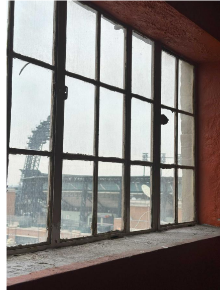
INTERIOR VIEW OF 5TH FLOOR WINDOW
