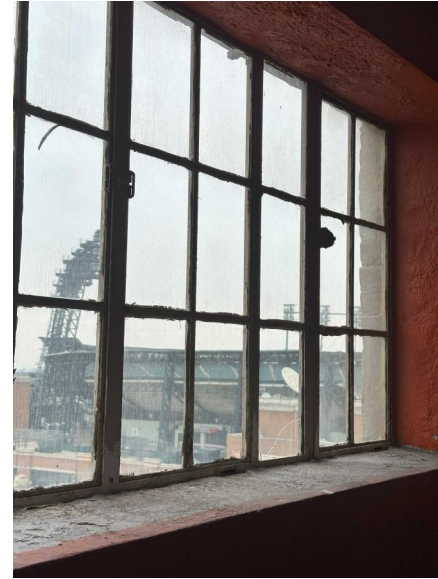
INTERIOR VIEW OF 5TH FLOOR WINDOW
