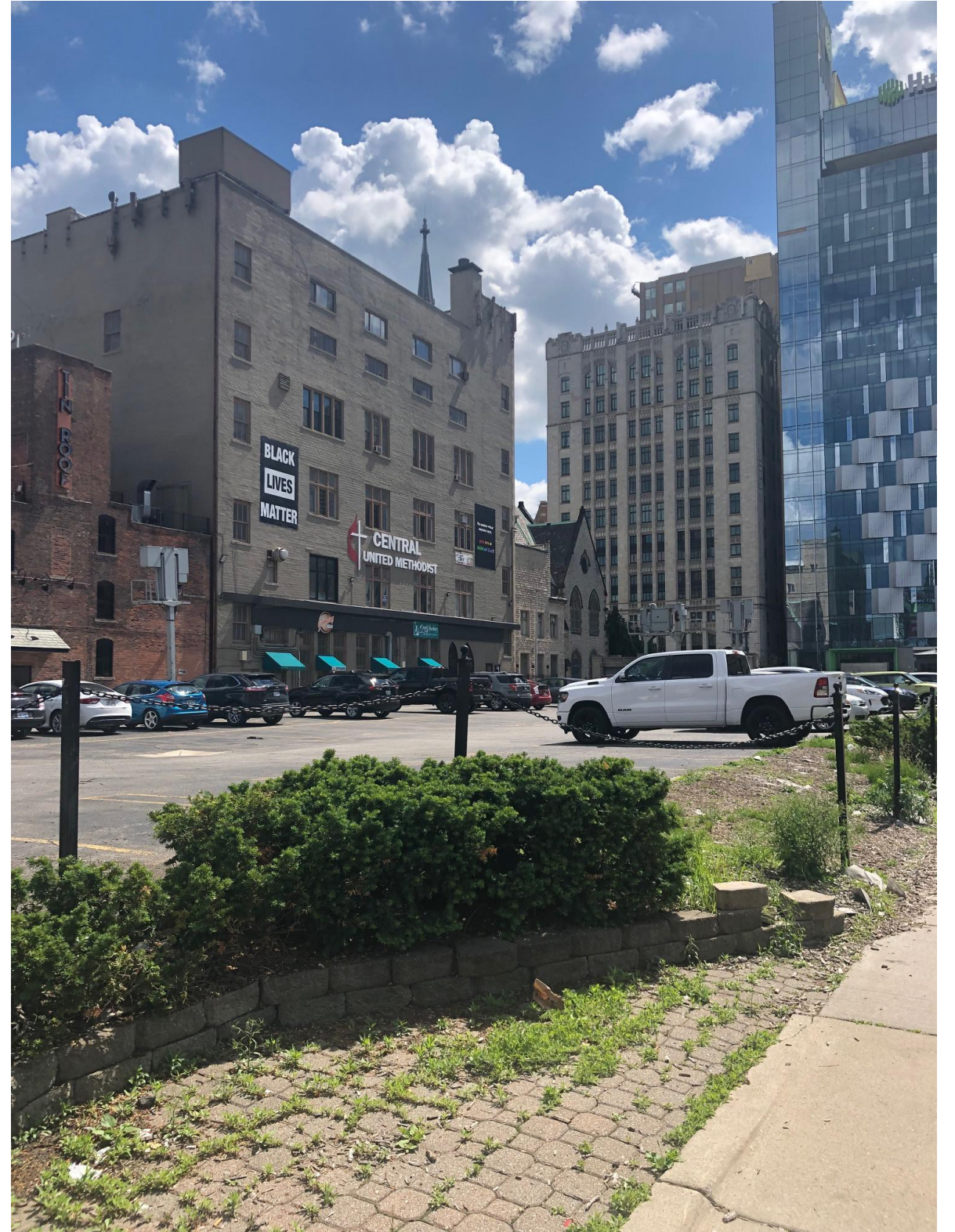
NORTH VIEW OF CHURCH HOUSE
