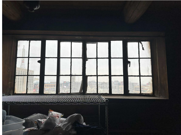
INTERIOR VIEW OF 5TH FLOOR WINDOW
