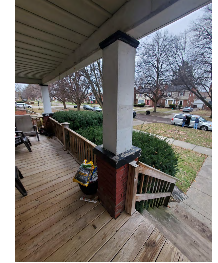
ON PORCH LOOKING SW
