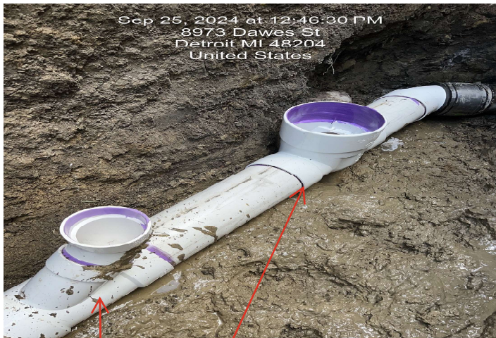
Clean Out & Backflow Valve Installation
