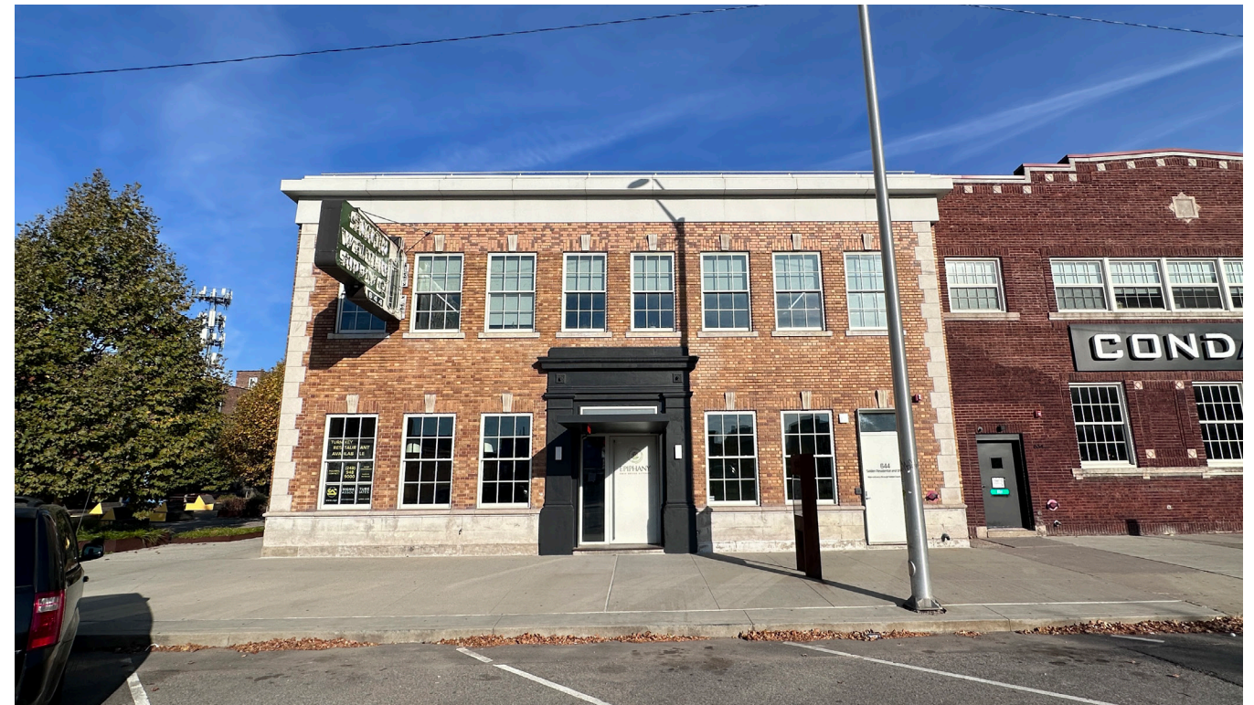
Looking North from Selden Street
