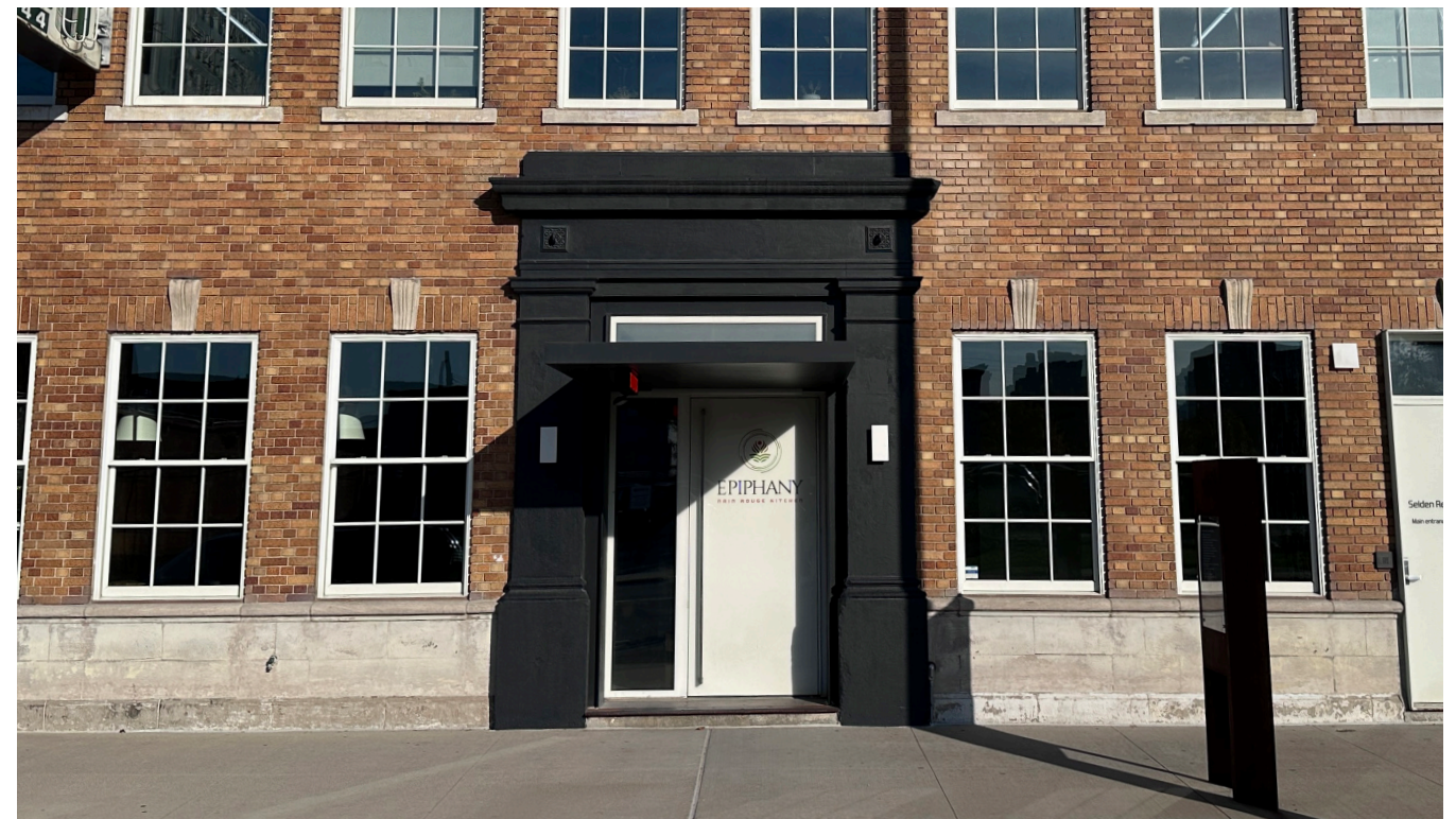
Looking North from Selden Street (existing painted limestone main entry; existing double hung aluminum frame windows w/ white frame)
