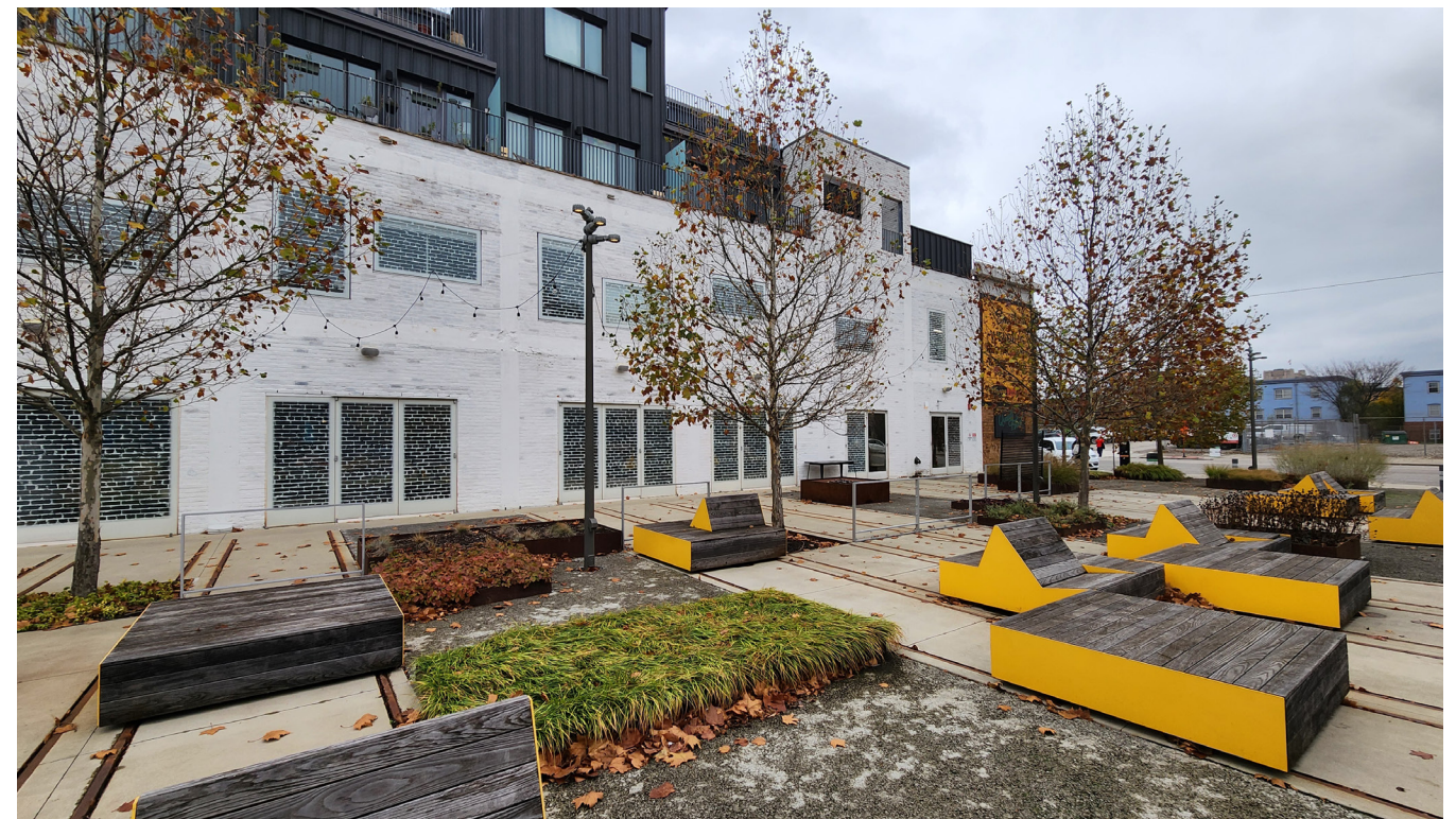
Looking East from courtyard (existing painted brick and glazing graphic detail; typical on 1st and 2nd floor West facade)
