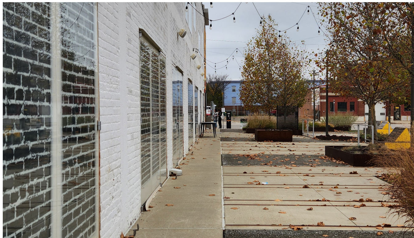
Looking South from courtyard (subject building on left; existing glazing graphic detail; typical on 1st and 2nd floor West facade)
