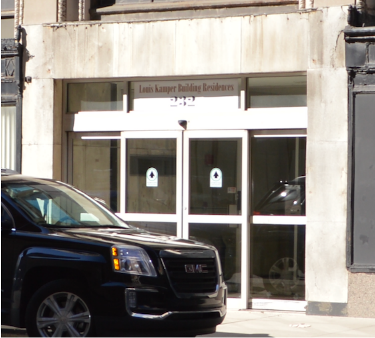
South building entrance, Sept. 2016
