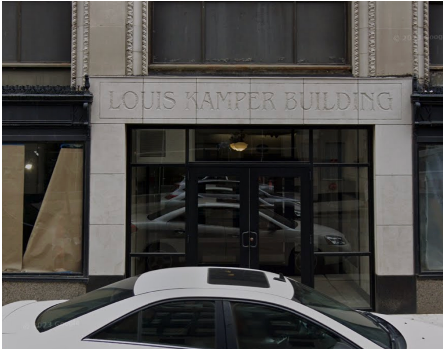
Oct. 2023 after work completed
