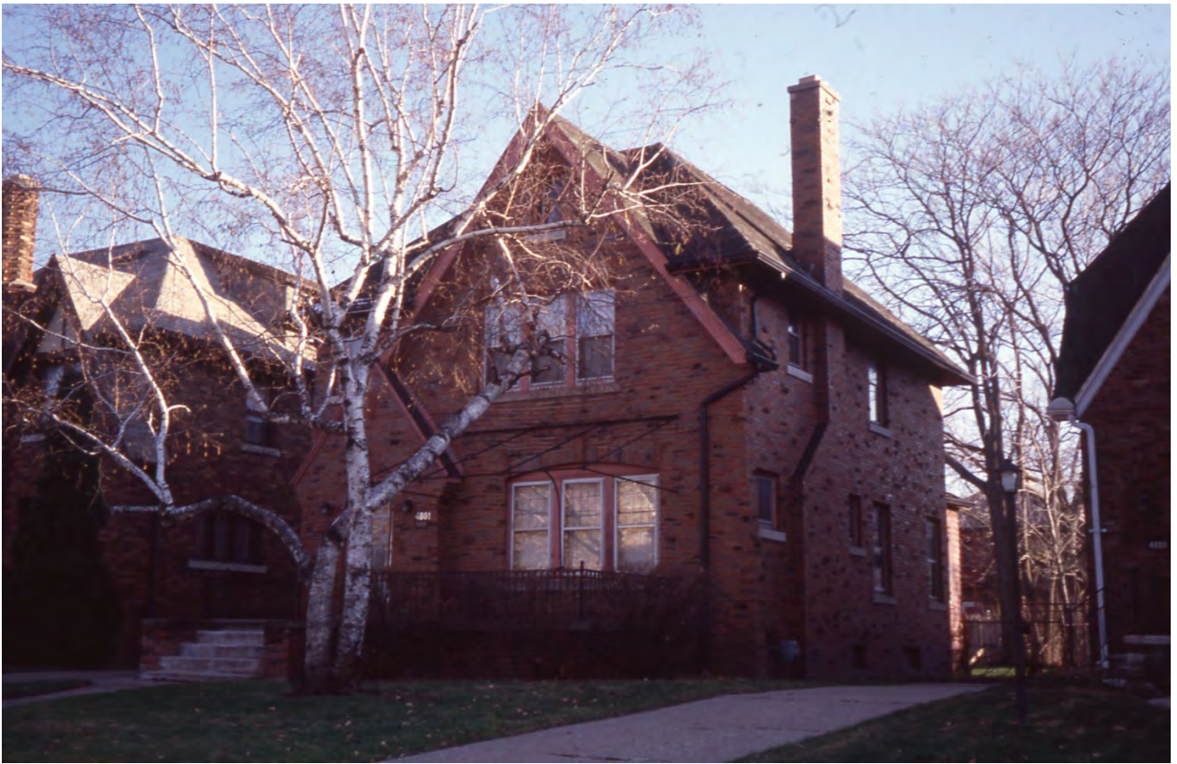
1999 Historic Designation Photo- Front Elevation
