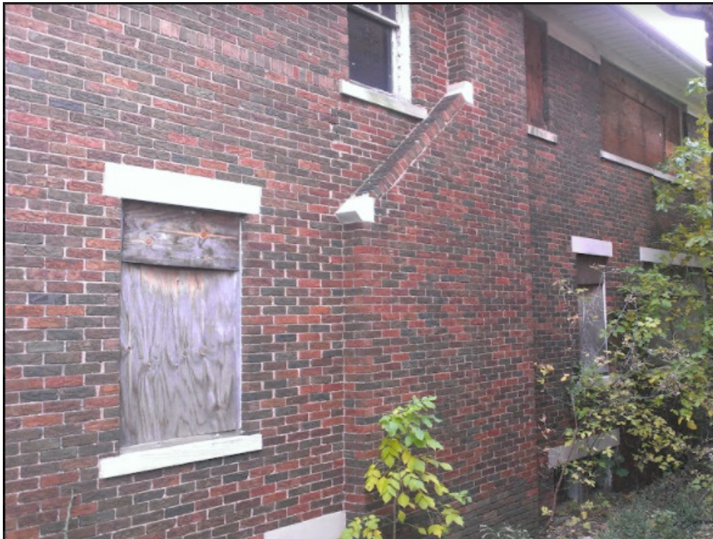
Original home as purchased (NOV 2014)– Left Side
