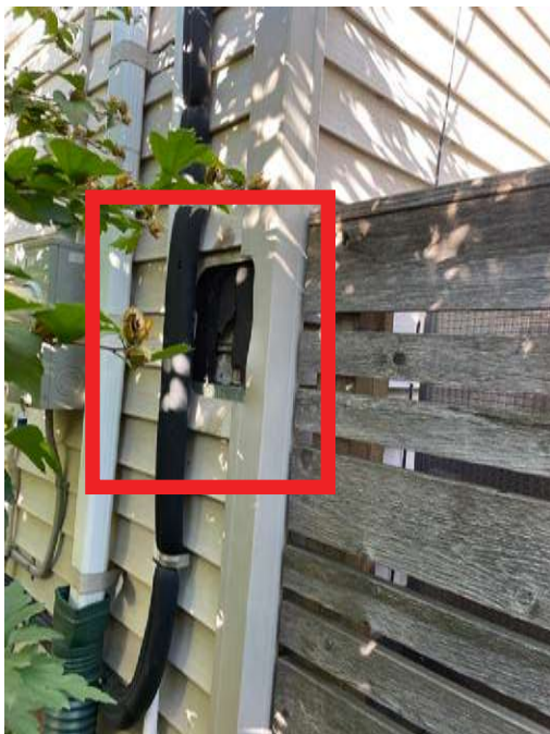
Measurement Location - Hole in non historic vinyl siding allowing access
