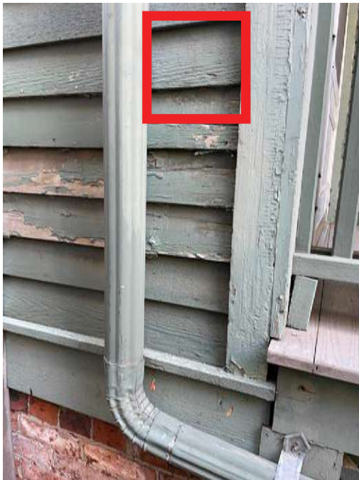
Measurement Location - Northeast (front) corner of house
