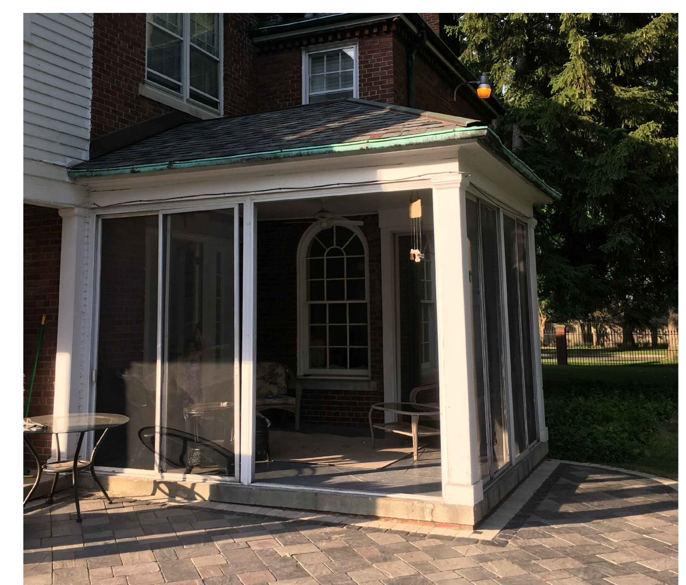
B EXISTING CONDITIONS PHOTOGRAPH SEE ELEVATION 1
