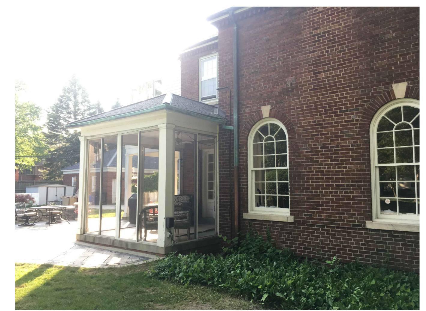
A EXISTING CONDITIONS PHOTOGRAPH SEE ELEVATIONS 2 AND 3
