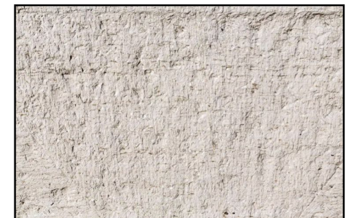
LIMESTONE SLAB - TRIM, BASE AND CORNICE
