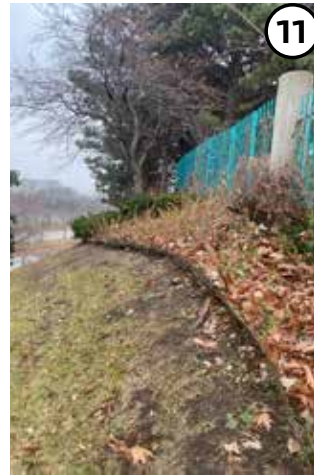
Reinstall landscape edging
