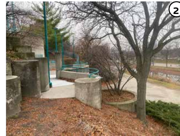
(1) Honeylocust tree and ornamental tree in planter are in good condition. Reset landscape edging, remove weeds from planing beds, add landscape fabric, topsoil, mulch, and ground cover. Reseed grass area leading up to sidewalk
