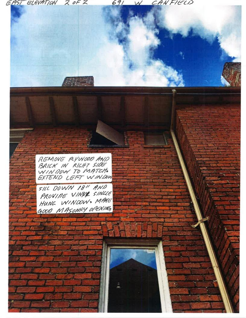
EAST ELEVATION 1 OF 2 691 W CANFIELD SUPPLY AND INSTAL NEW VINYL SINGLE HUNG WINDOW TO MATCH BESIDE. MAKE GOOD REMOVE SECURITY GRIC REMOVE EXISTING GLASS BLOCK AND PLYWOOD AT BASEMENT WINDOW, LOWER SILL 18" WINDOWS PROVIDE OPERATE AND PROVIDE NEW VINY EXISTING OPENING SINGLE HUNG WINDOW.
