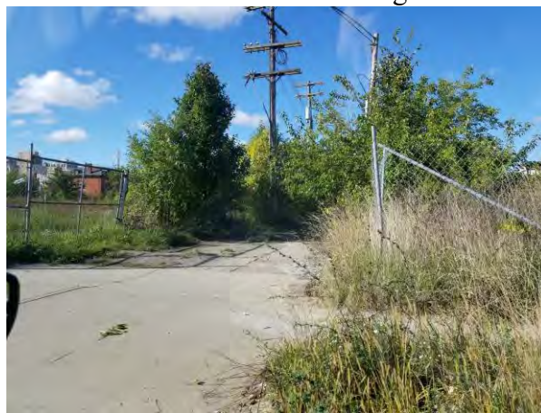
Site along Brush Street and Public Alley – 10/04/19
