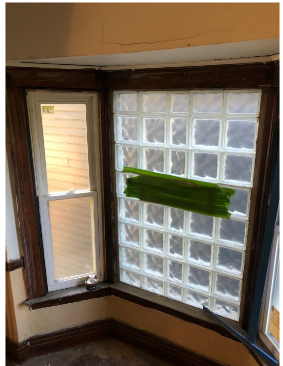
Windows J & K (Interior)
