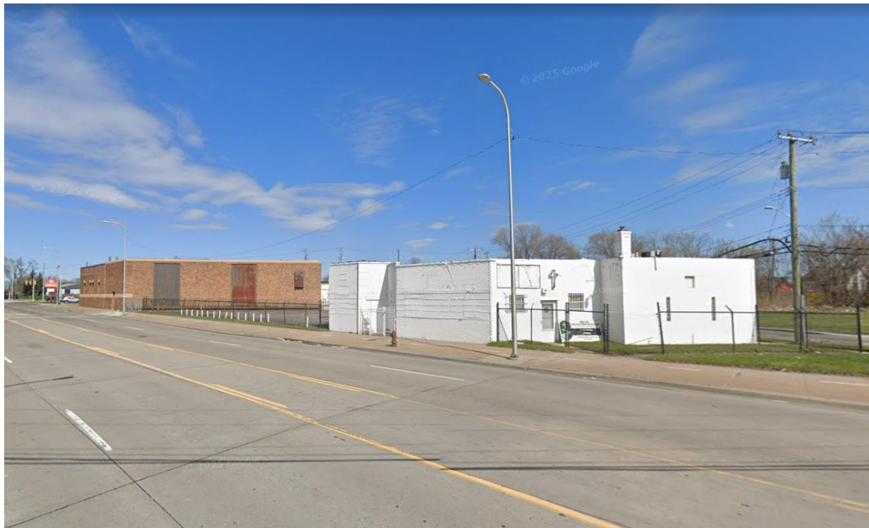
Existing conditions of 4850 and 4900 Conner
