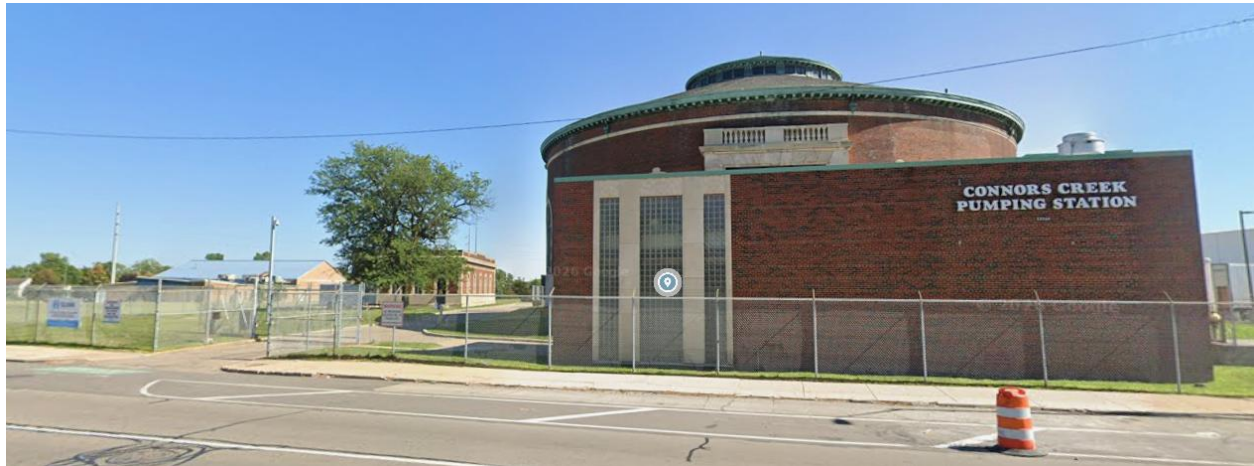
July 2025 Google Streetview of existing Conner Creek Pumping Station at 12264 E. Jefferson.
