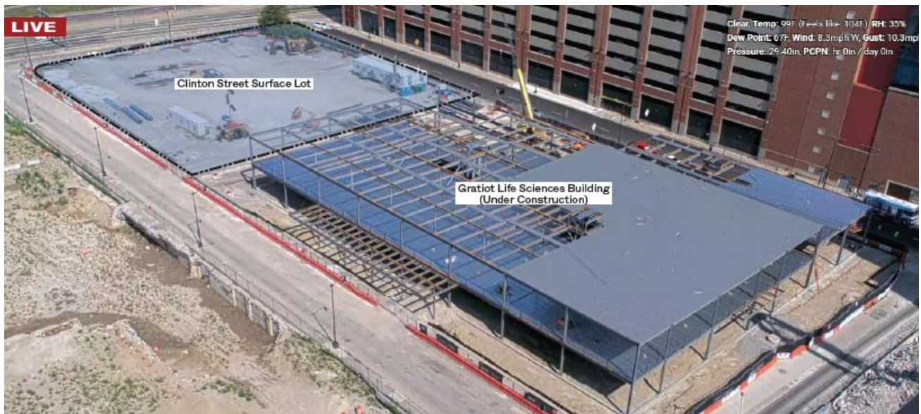
Photo of Gratiot Life Sciences Building under construction
