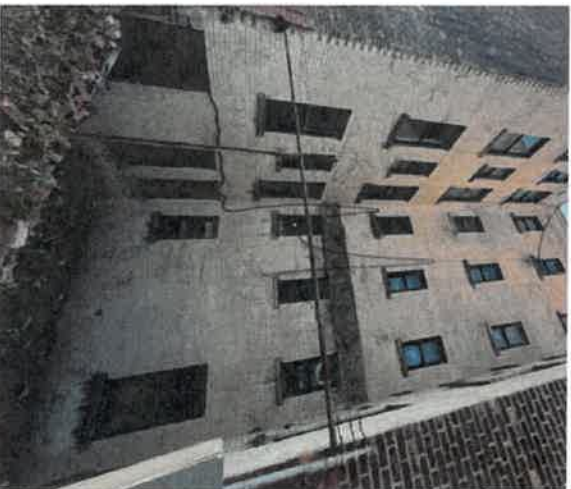
Weathered brick was surface coated in mortar and not salvageable. Repaired with CMU block for durability. Entire interior area to be painted and hide CMU block.
