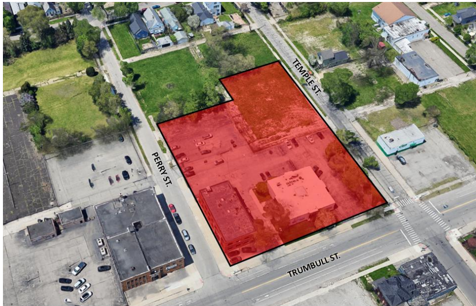
Existing site as viewed from an aerial perspective.
