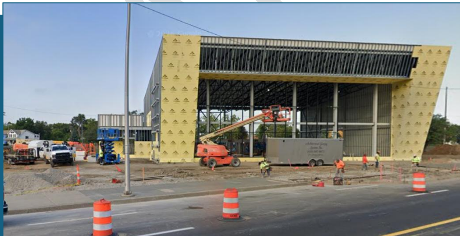
MERIT PARK – UNDER CONSTRUCTION
