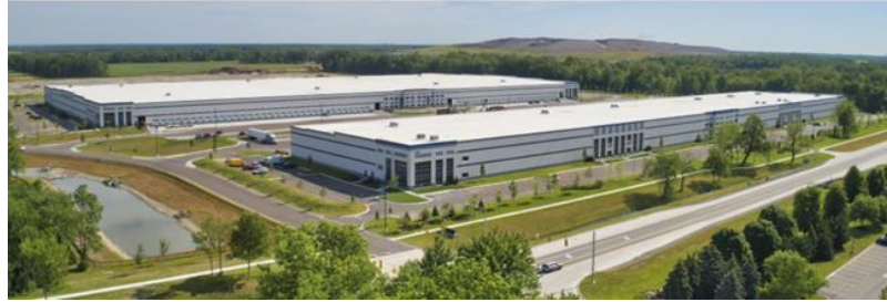
Crossroads Distribution Center – Van Buren Township, MI
