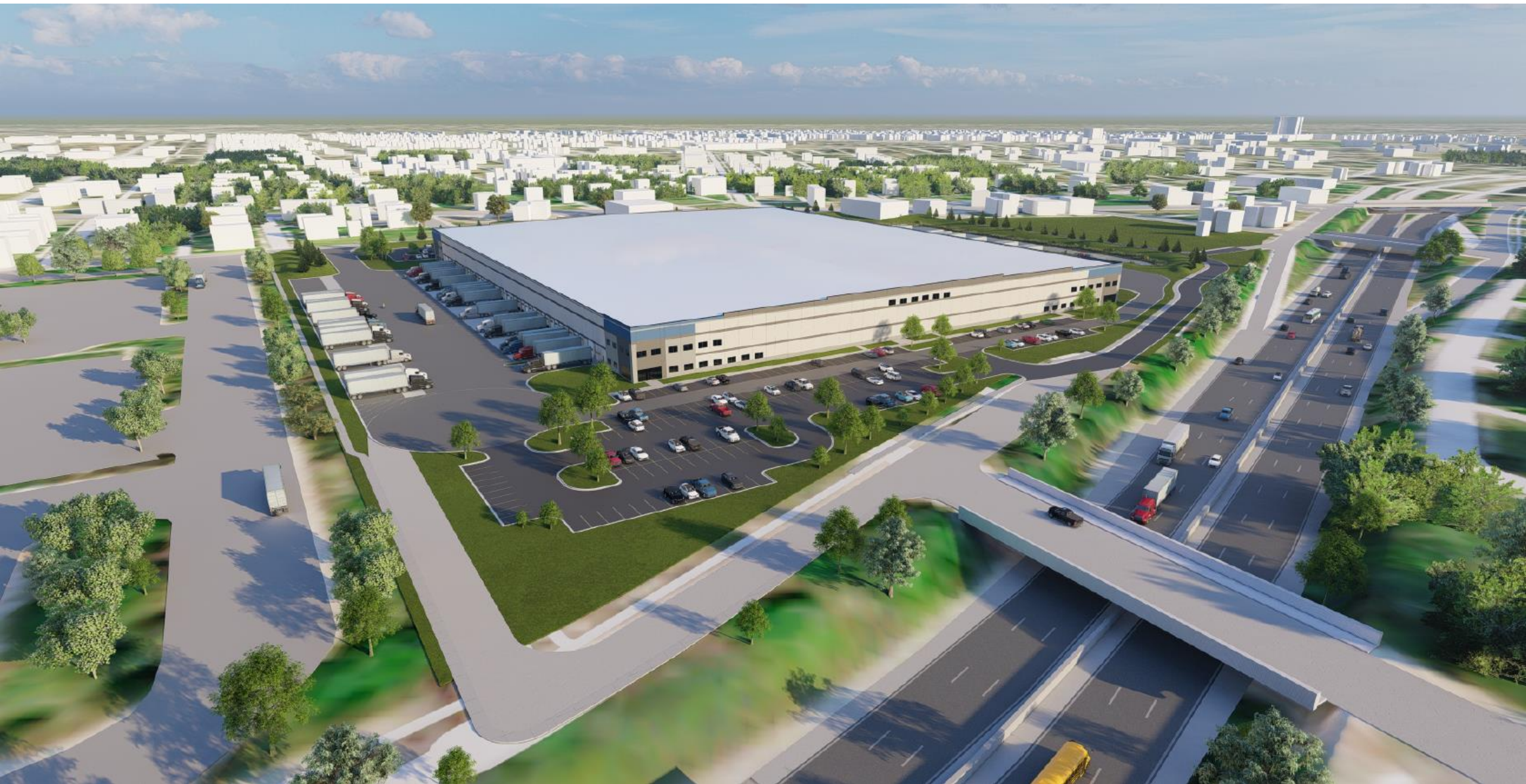
Facility View Looking Northeast from I94
