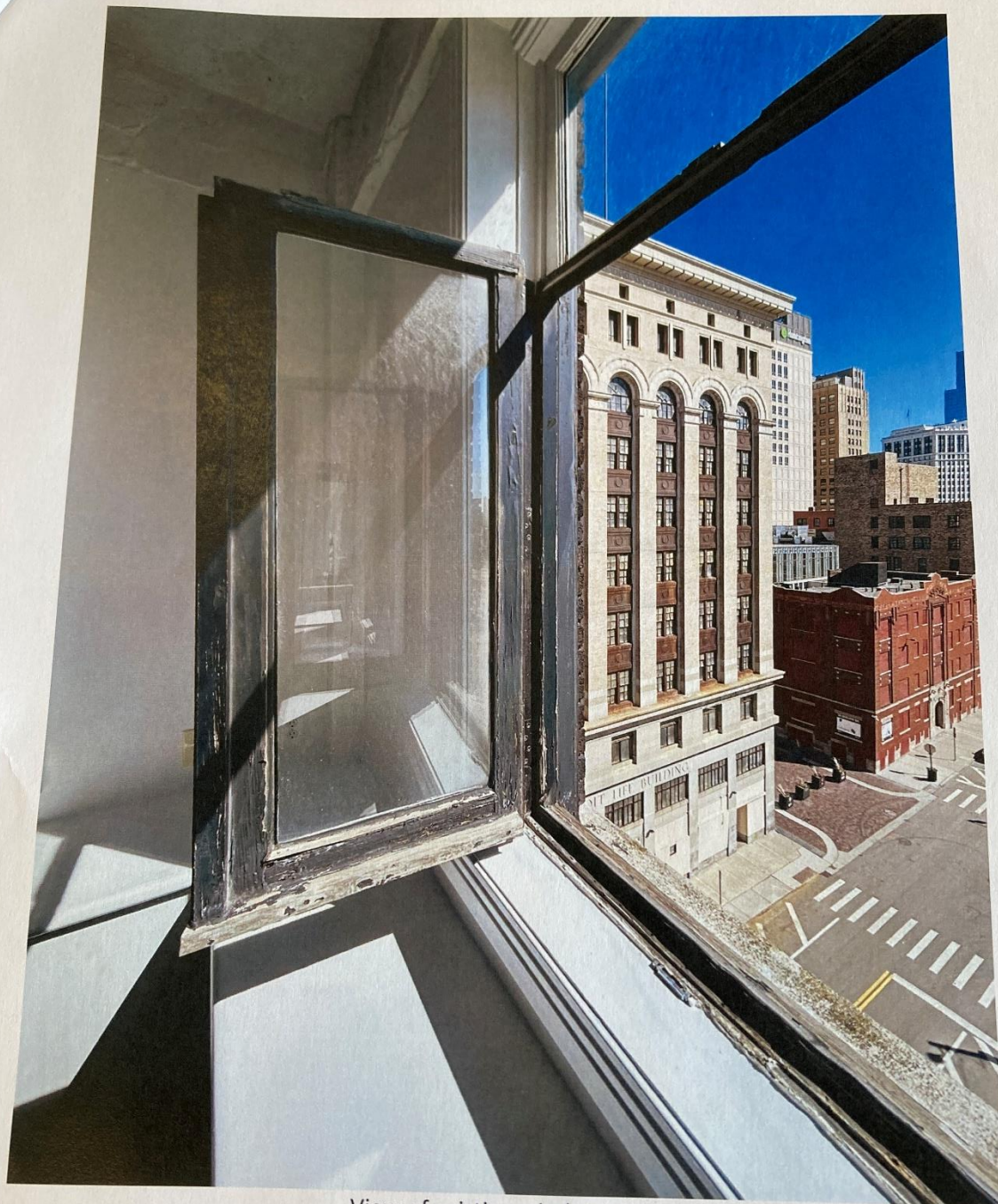
View of existing window sash
