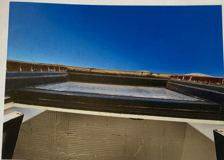
Window frame head and transom above
