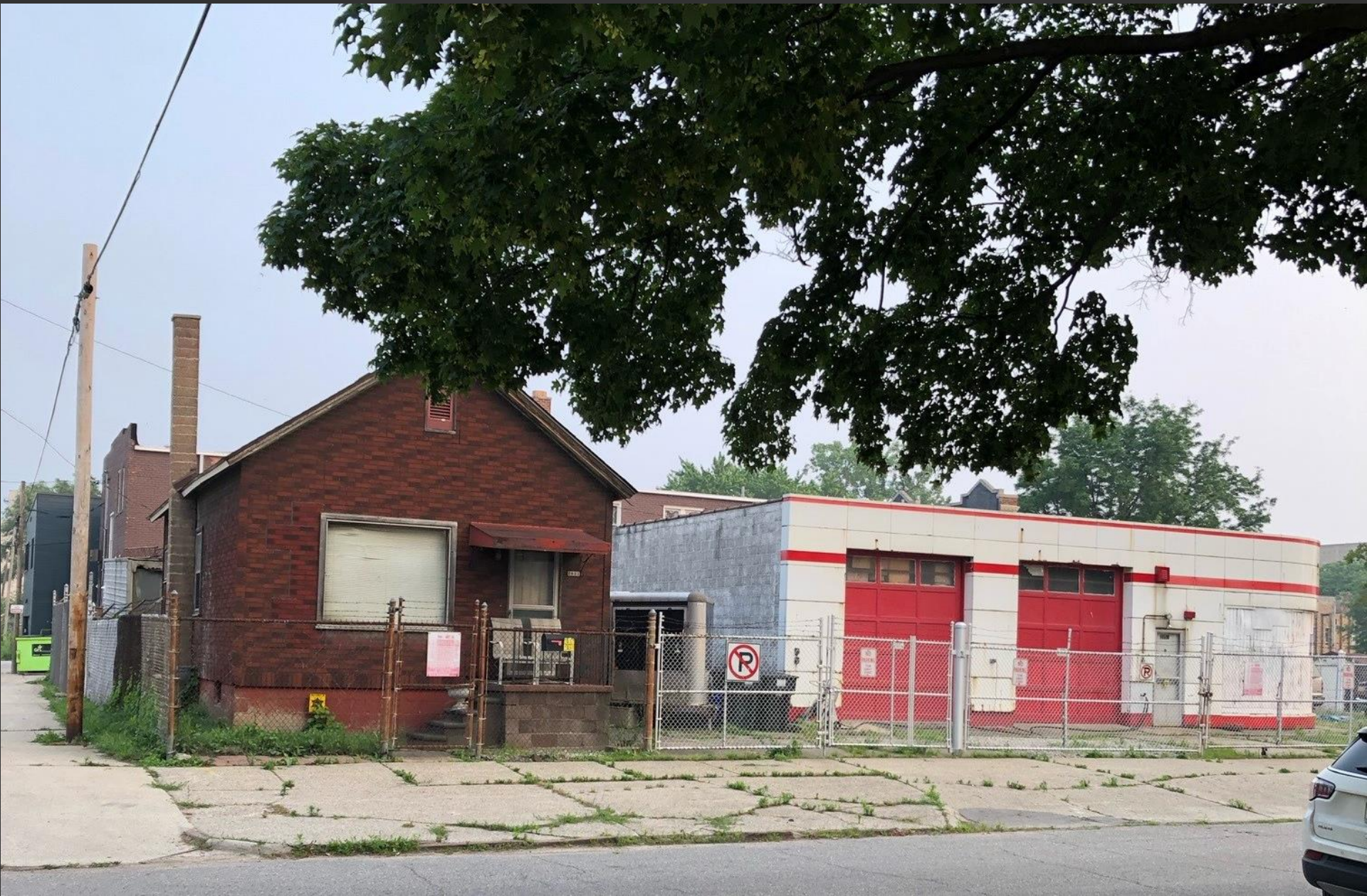
Adjacent properties across alley to west
