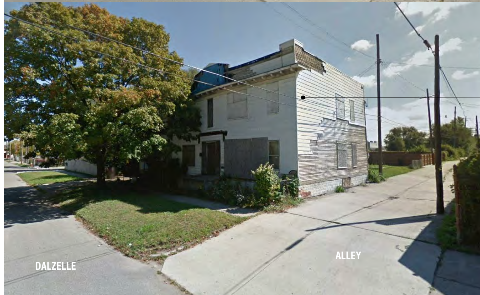
PREVIOUS 4 UNIT APARTMENT BUILDING ON SITE
