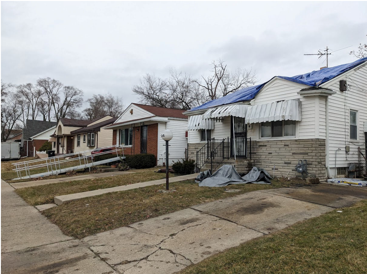
View of east side of Fenelon Street looking north, between Stockton and East Hildale Streets. All photos included in this report were taken by historic staff on January 5, 2023 within the proposed district.
