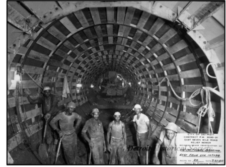
Detroit Historical Society photo of the Michigan Sewer Construction Company workers at E. 7 Mile Relief Sewer.
