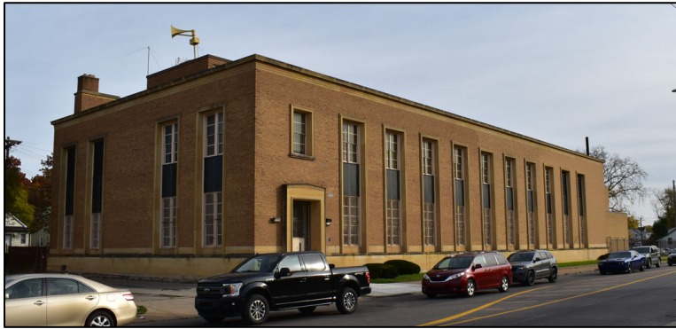
The AT&T/Michigan Bell Telephone Exchange building - 18862 Ryan Road (1941 and additions)
