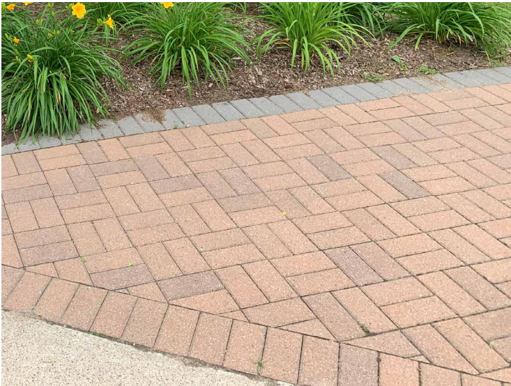
CLOSE-UP OF EXISTING BRICK PAVERS TO BE SALVAGED AND REUSED ONSITE
