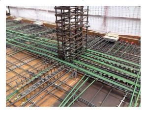
FIGURE 2: POST-TENSIONED SLAB CONSTRUCTION
