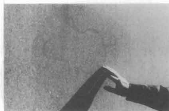
Figure (b) Most of the image was removed using a rag saturated with a mixture of solvents, including acetone, lacquer thinner and N-methy-2-pyrrolidone.
