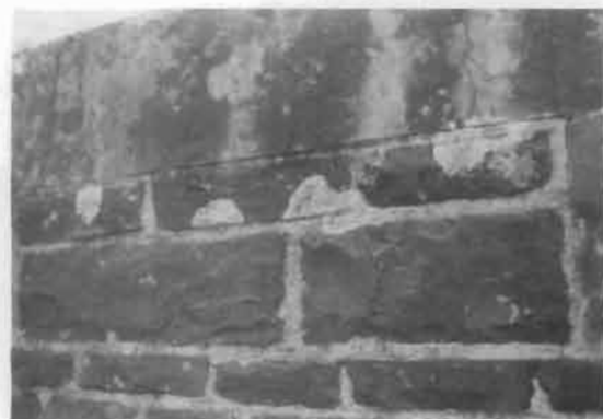
Figure 20. Plant growth such as lichens growing on a protected side of this limestone and granite parapet wall, can be damaging even to a relatively hard stone like granite because lichens secrete oxalic acid. Lichens can usually be removed, after soaking with water by scrubbing with a stiff natural bristle brush.
