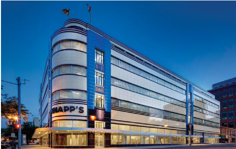
[7] (a) J.W. Knapp's Department Store, built 1937-38, in Lansing, MI, was constructed with a proprietary material named "Maul Macotta" made of enameled steel and cast-in-place concrete panels. Prior to its rehabilitation, a building inspection revealed that, due to a flaw in the original design and construction, the material was deteriorated beyond repair. The architects for the rehabilitation project devised a replacement system (b) consisting of enameled aluminum panels that matched the original colors (c). Photos and drawing (a-b): Quinn Evans Architects; Photo (c): James Haefner Photography.
