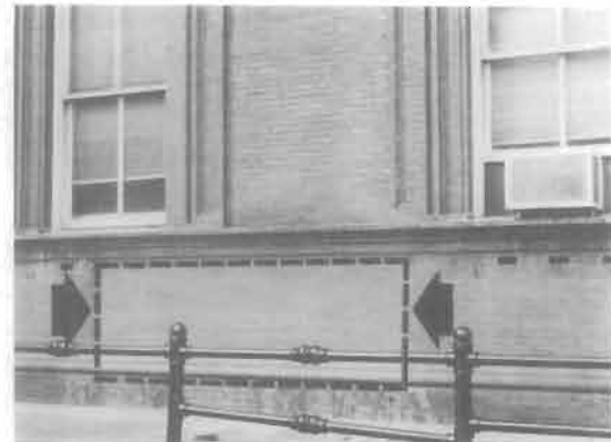
Figure 9. A test patch on brick to remove a century of dirt reveals only a slight difference in appearance between the cleaned and the uncleaned brick. The hard-baked outer skin of the brick provides a surface that is not only impervious to dirt penetration, but resists dirt accumulation. Photograph: Christina Henry
