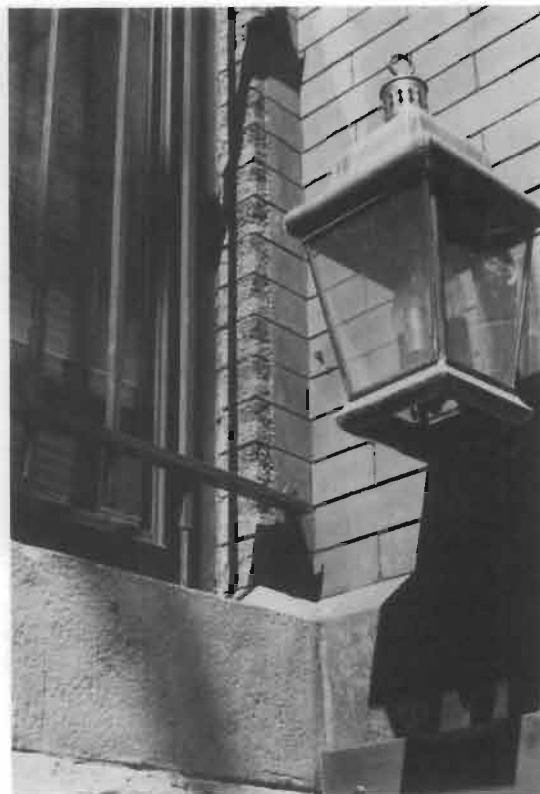
Figure 27. Heavily pitted by sandblasting, this window recess provides a vivid contrast to adjacent un-damaged brick protected from abrasion by a metal signboard.
