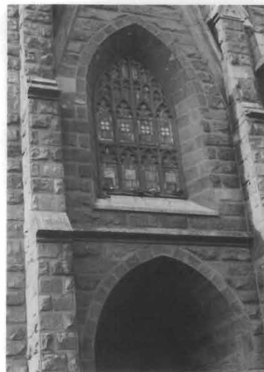
Figure 28. If water, or water and detergent wash, does not remove the pigeon droppings from this sandstone sill and stringcourse below, it may be necessary to use a dilute acidic cleaner containing hydrofluoric acid, providing the sandstone is not calcareous and thus, acid-sensitive.
