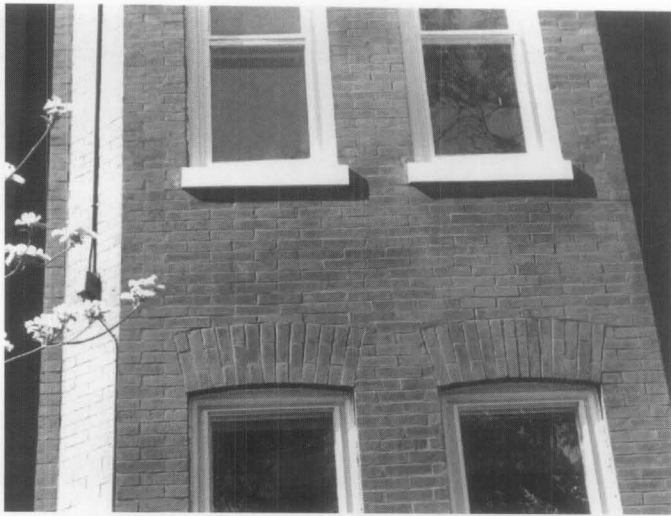
Figure 24. Although the application of a water-repellent coating was probably not needed on either of these buildings, the coating on the brick building (above), is not visible and has not changed the character of the brick. But the coating on the brick column (below), has a high gloss that is incompatible with the historic character of the masonry.
