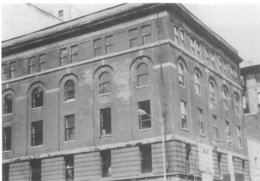
Figure 26. Efflorescent salts appearing on many of the brick piers of this turn-of-the-century building may indicate the existence of clogged interior gutters that, because they no longer function have been supplemented by an exterior rain removal system. Photograph: National Park Service
