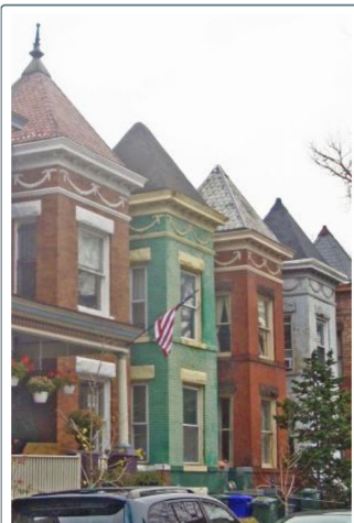
In this row of late-nineteenth century brick rowhouses, the painted brick shows signs of efflorescence (second from left) and flaking (r).
