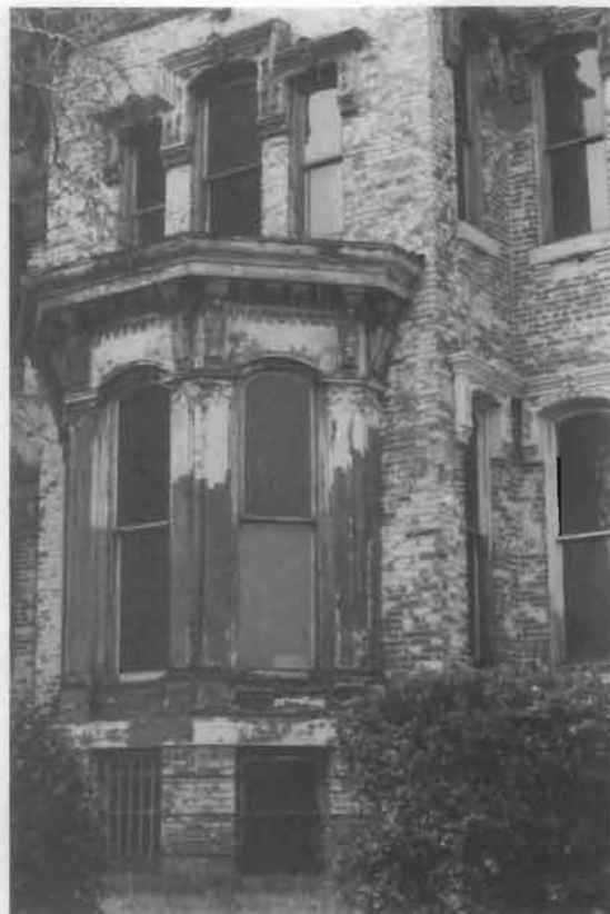
Figure 3. Know what you are cleaning. If the painted surfaces of the projecting bay window on this once elegant Second Empire brick mansion were still intact, it would not be easy to identify the beltcourse as sandstone, the windows and window frames as wood, and the cornice and all of the window hoods as pressed metal. Cleaning so many different building materials may require a variety of techniques and treatments.
