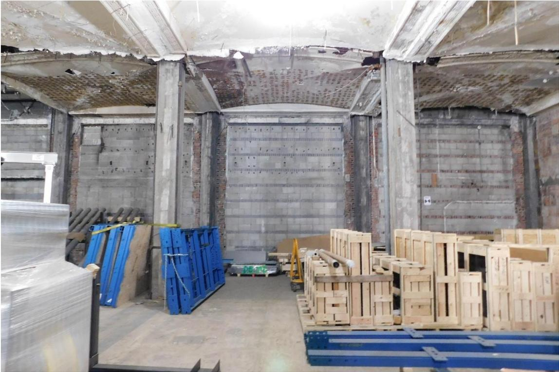
Figure 56: Interior, Looking West, CMU Infill Where Alley Storefronts used to be located.
