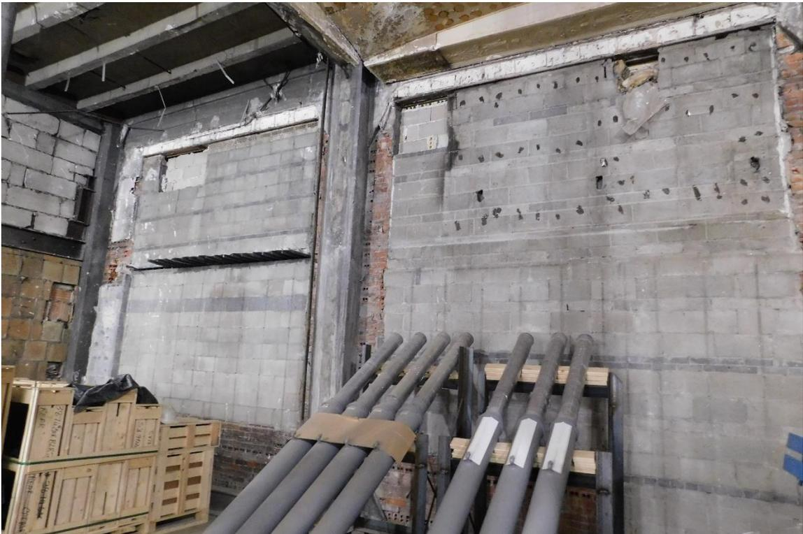
Figure 57: Interior, Looking West, CMU Infill Where Alley Storefronts used to be located.
