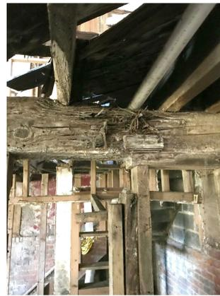
BASEMENT - BEAM - WATER DAMAGE
