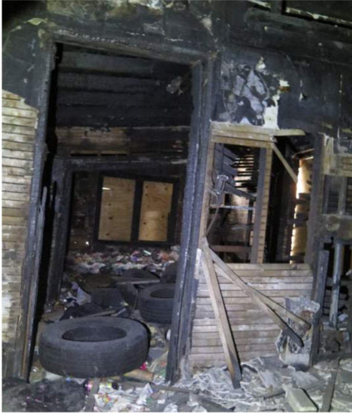
Figure 10 Wood Stud Walls with Extensive Fire Damage
