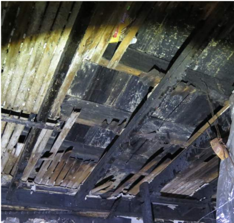
Figure 11 Second Floor Joist Framing with Extensive Fire Damage
