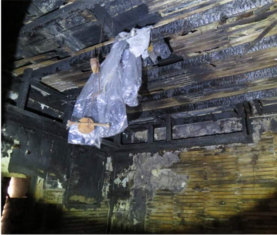
Figure 9 Second Floor Framing with Extensive Fire Damage
