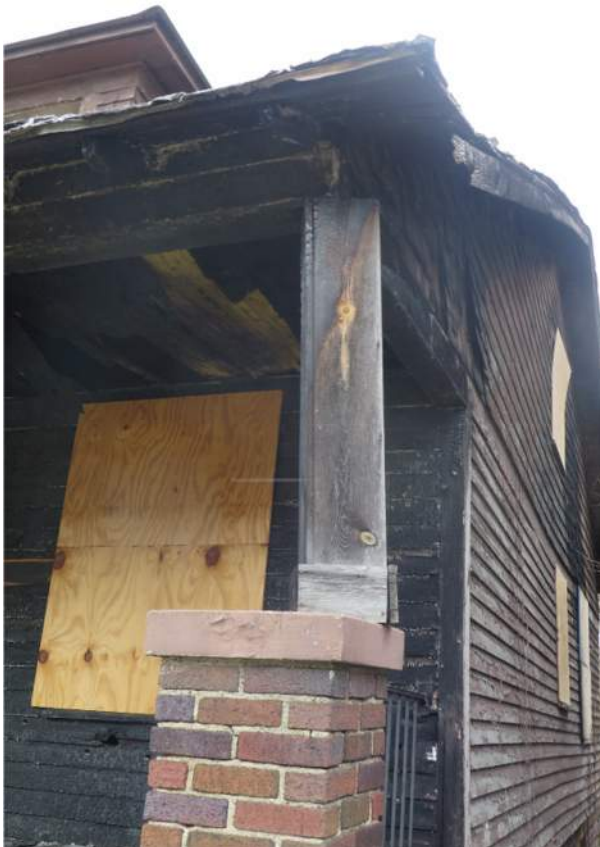
Figure 17 Wood Post Roof Support Out of Alignment
