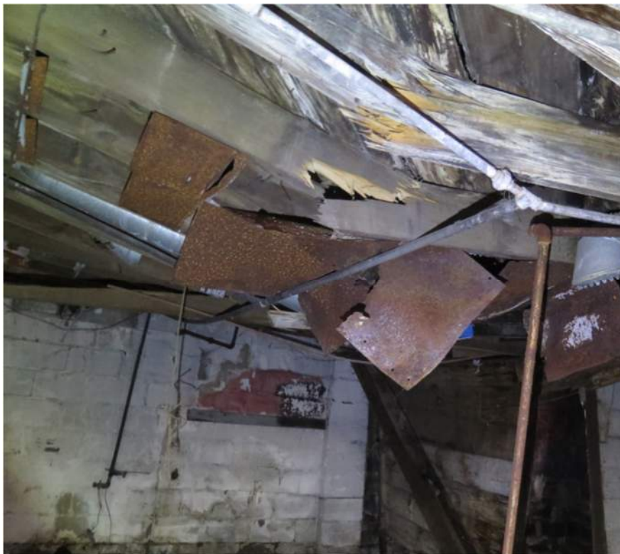
Figure 6 First Floor Failed Joist Framing
