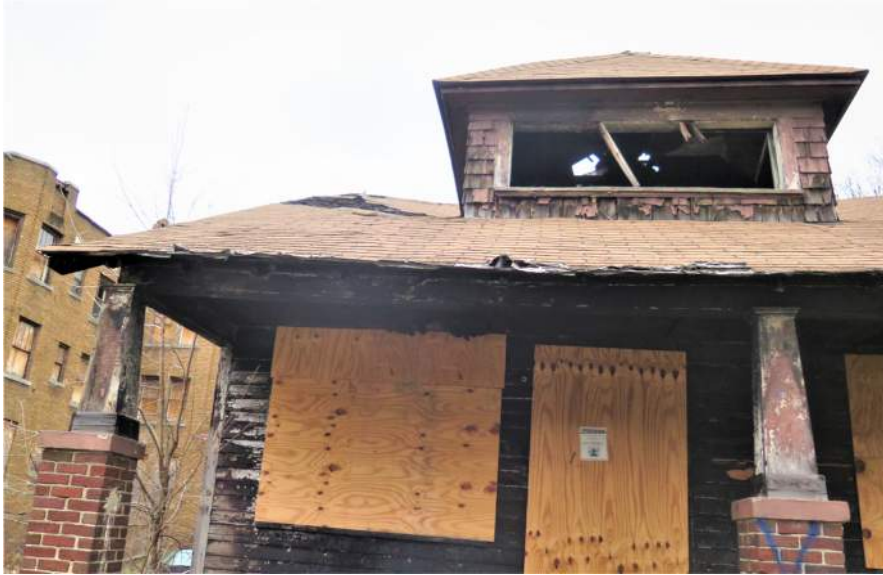
Figure 16 Apparent Sagging of Roof and Spandrel Beam
