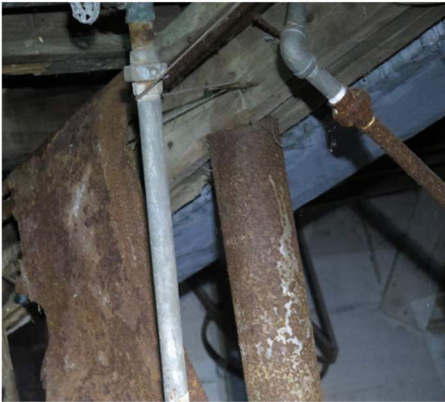
Figure 8 Apparent Punching Failure of Post Through Timber
