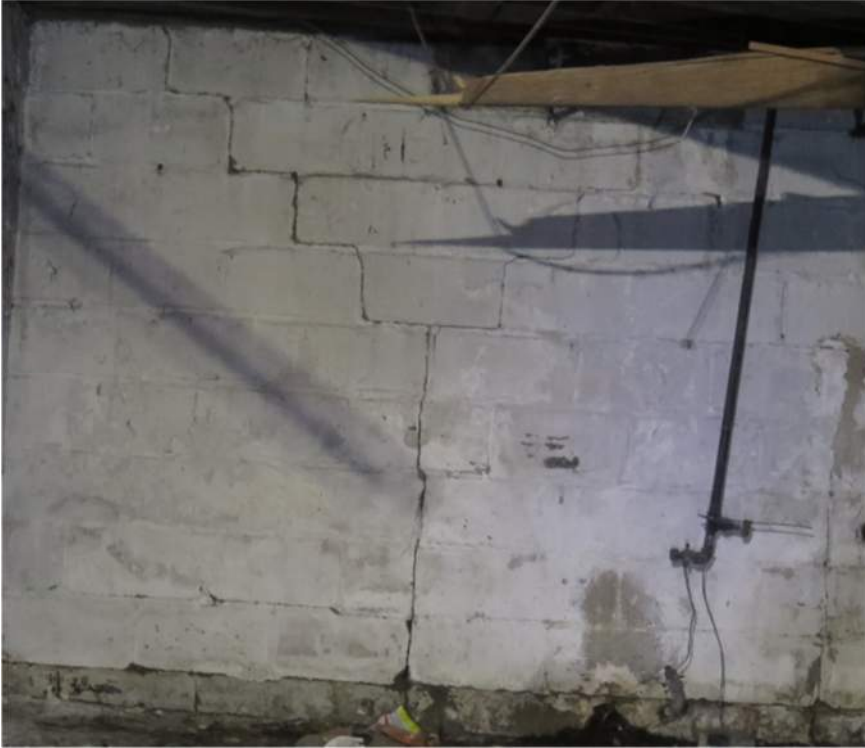
Figure 3 Existing Condition of Foundation CMU Walls With Cracking Observed
