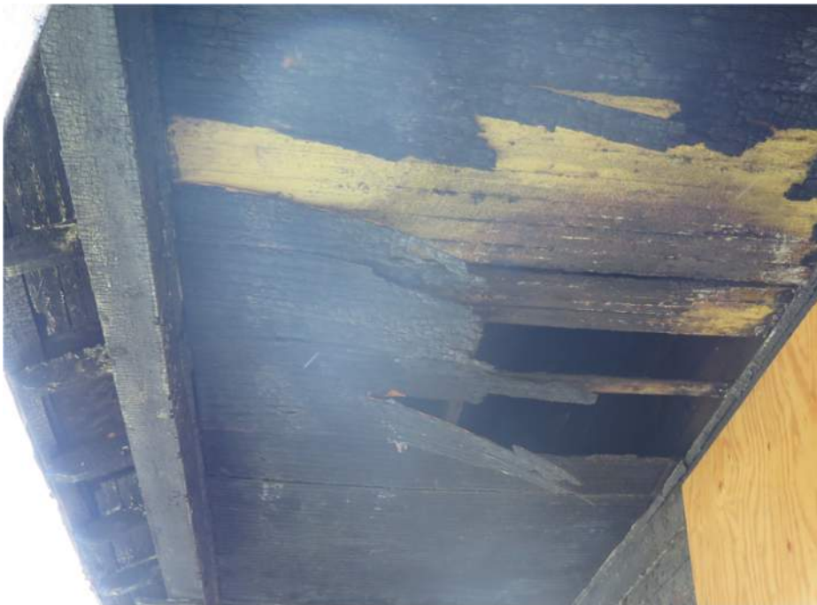
Figure 15 Underside of Porch Framing with Extensive Fire Damage
