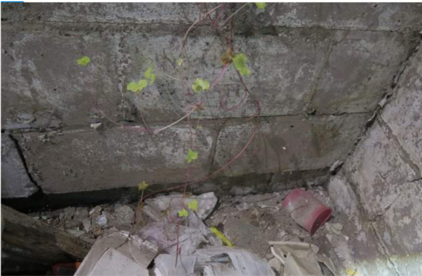
Figure 4 Vegetative Growth Through Foundation Walls
