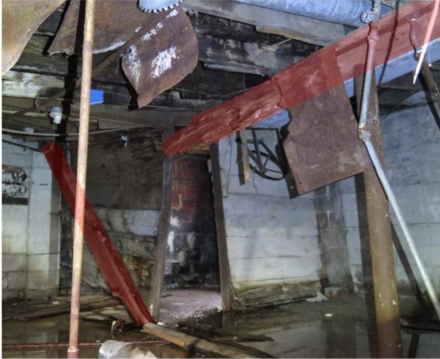
Figure 7 First Floor Failed Central Timber (Red)
