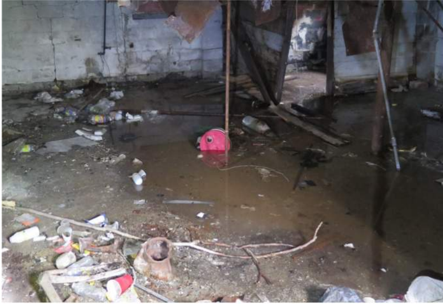
Figure 5 Basement Slab with Standing Water Observed
