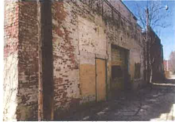
Photo 2: A view of the east side of the subject property.
