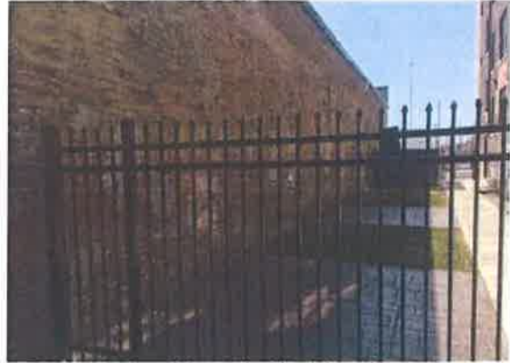
Photo 4: A view of the north side of the subject property.
