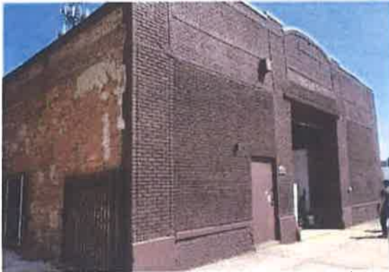
Photo 1: Looking southeast toward the subject building.
