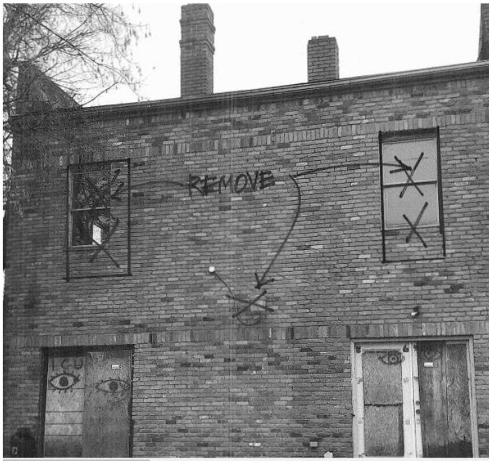
4114/4116 Trumbull Alteration of window opening by cutting into brick
