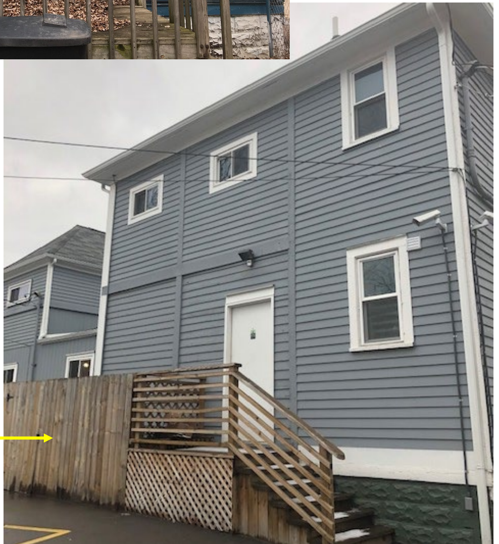
Wood fence enclosure – installed in place of free-standing CMU enclosure.
