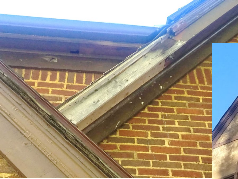
Wrap Wood Fascia, Soffits, Horizontal trim at edge of stucco gables, and double-hung window casings with Dark Brown Aluminum - Page Three
