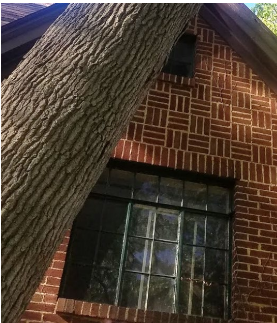
Original Windows – additional photos supplied by applicant
