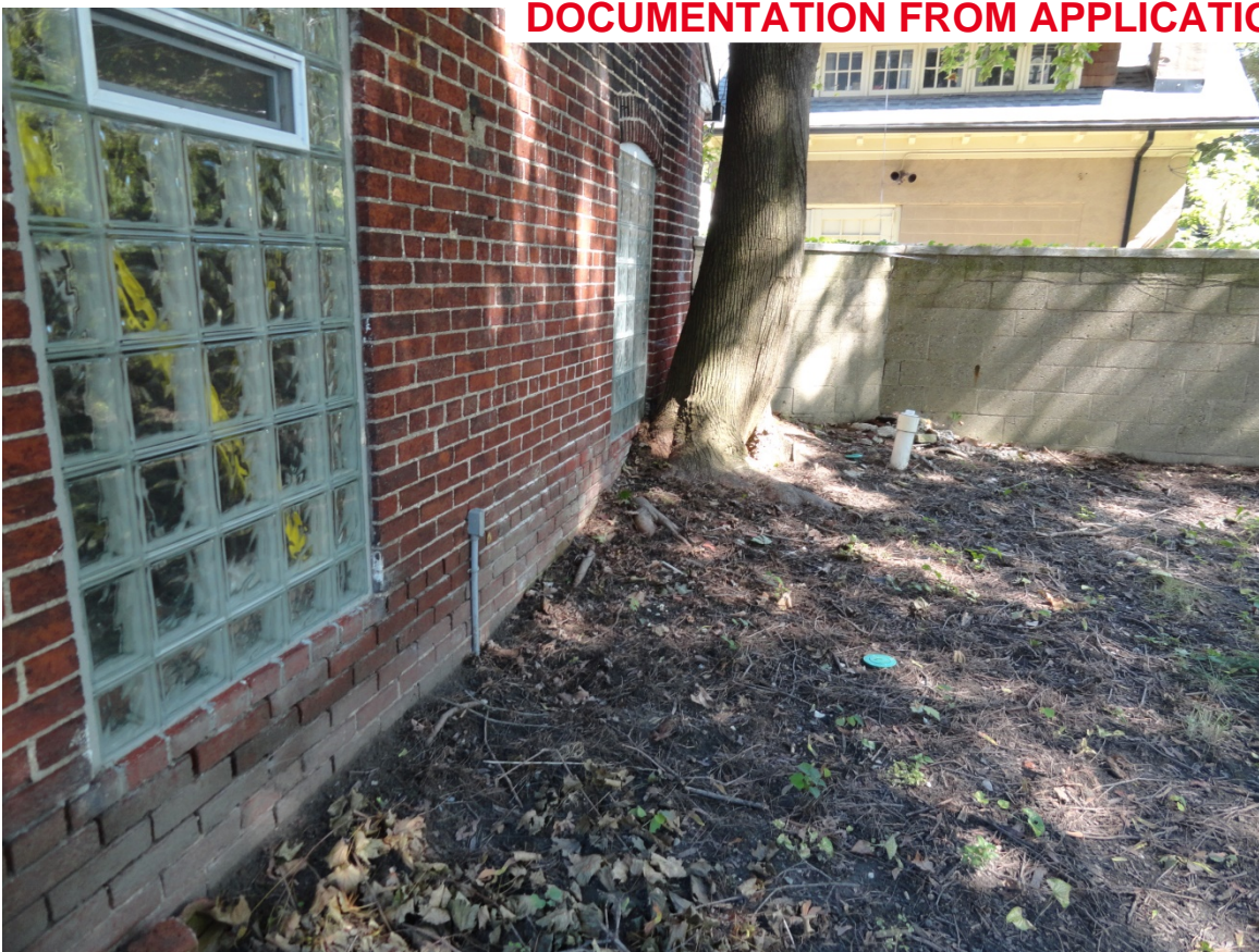
5-South Elevation Tree Encroachment
