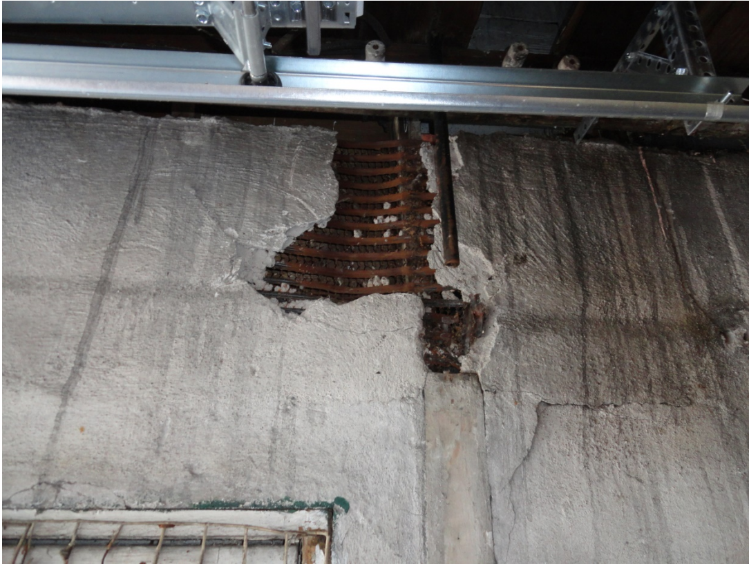
13- Interior wall deterioration at shed addition
