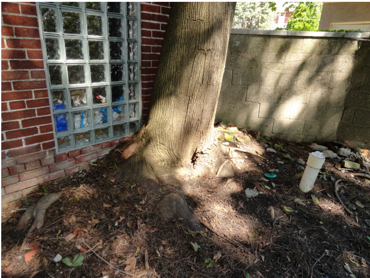
6-South Elevation Tree Encroachment
