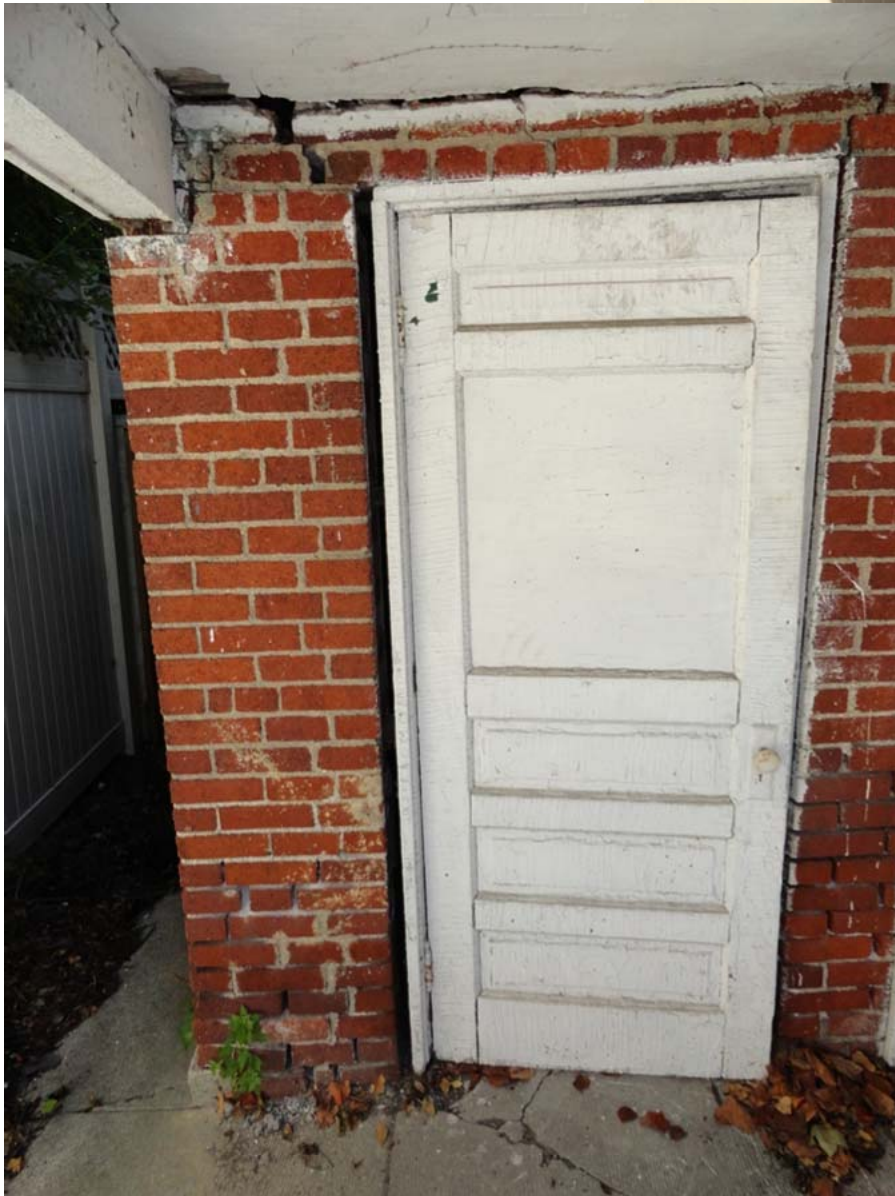
16- Shed Addition structural issue
