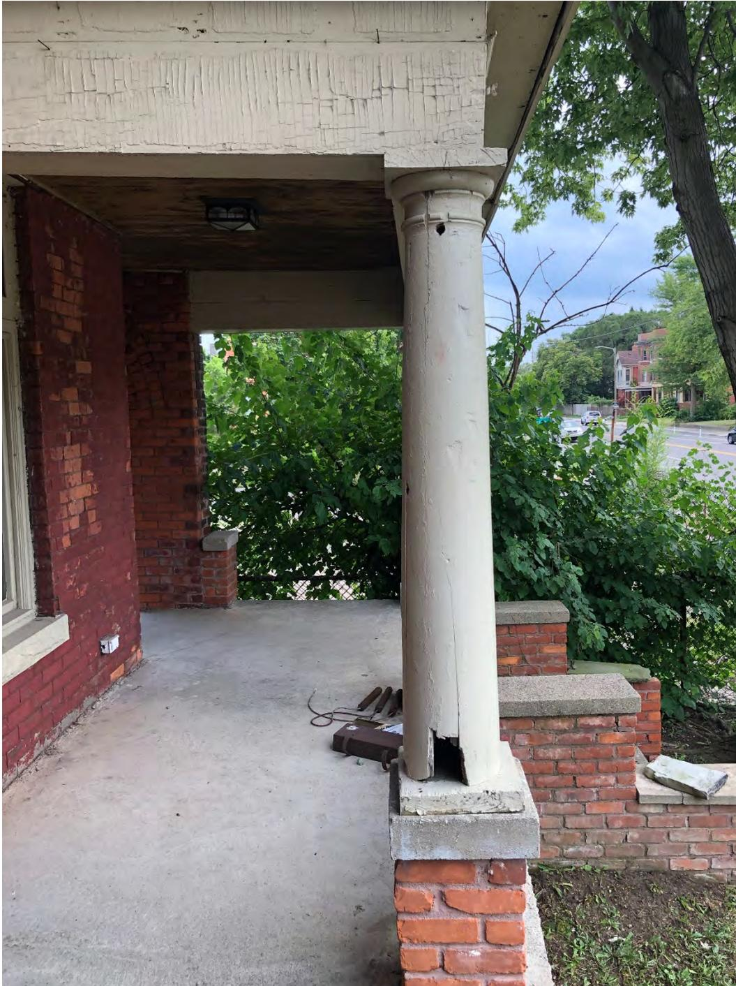
Detail image of wood damage at 4114 porch
