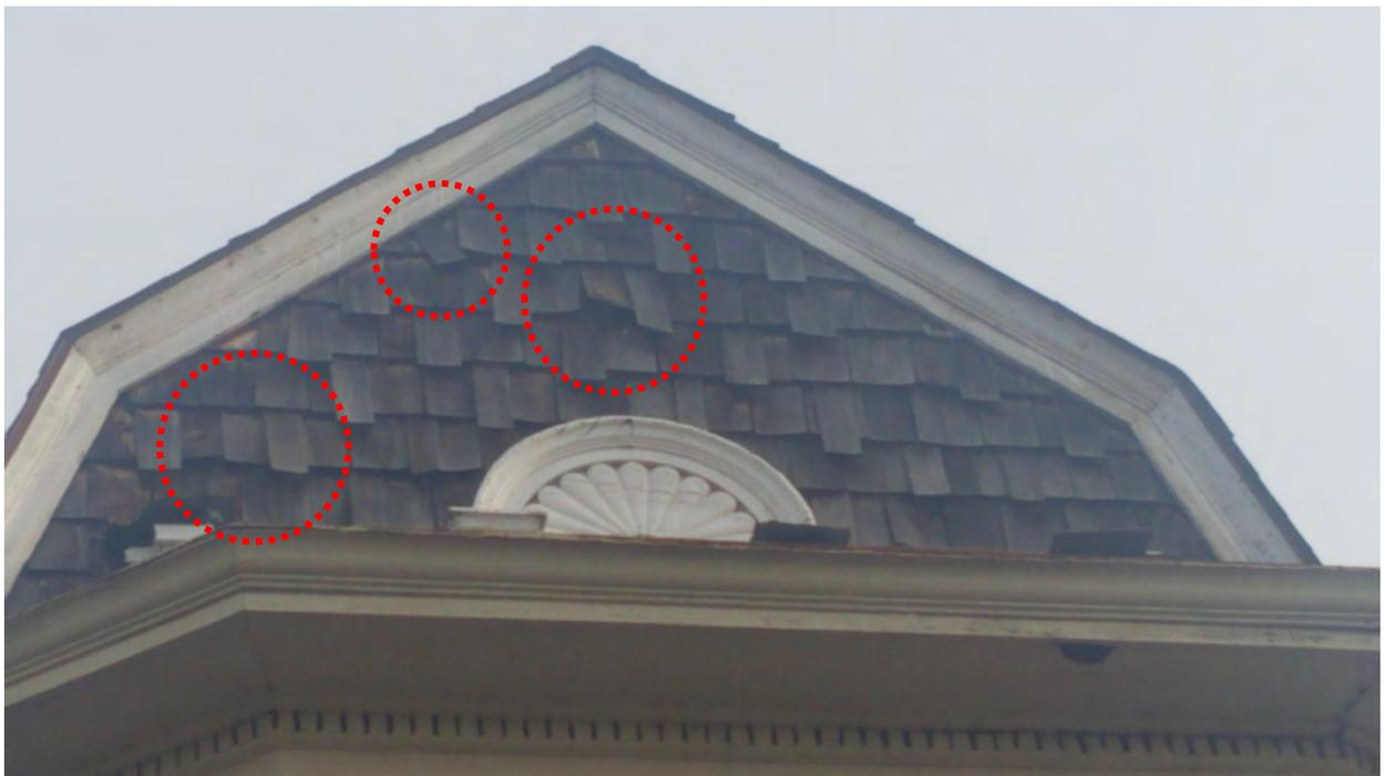
Dormer 1 (West Elevation) Identified are shakes with excessive curling or have become loose.
