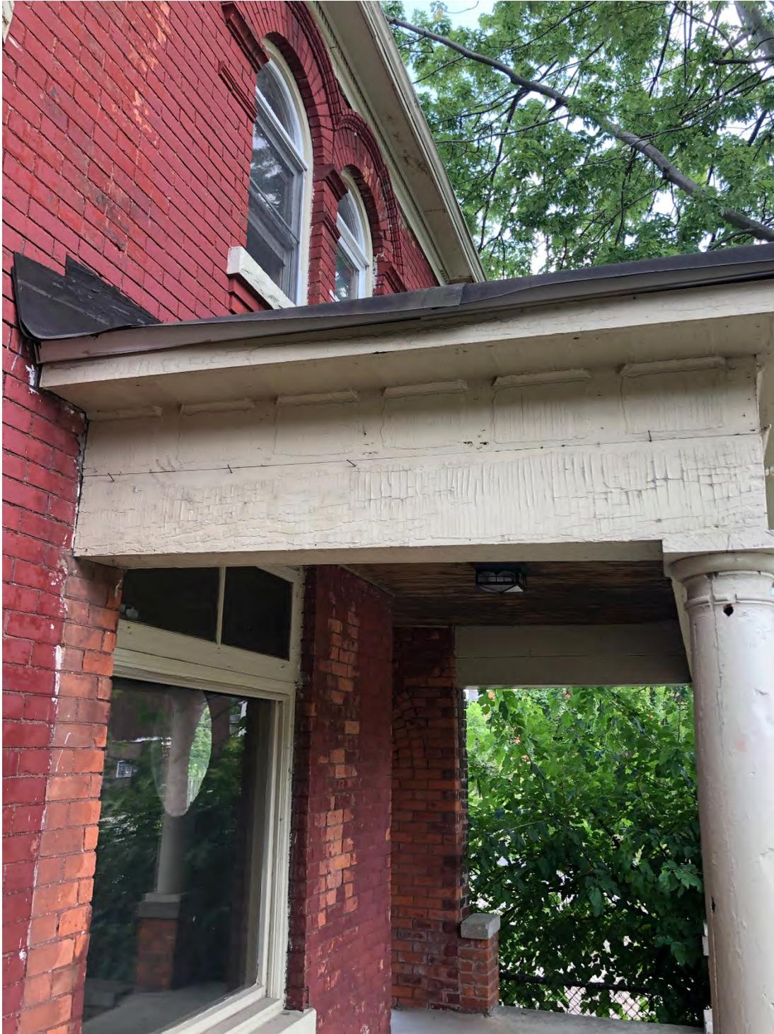
Detail image of typical wood damage at porch
