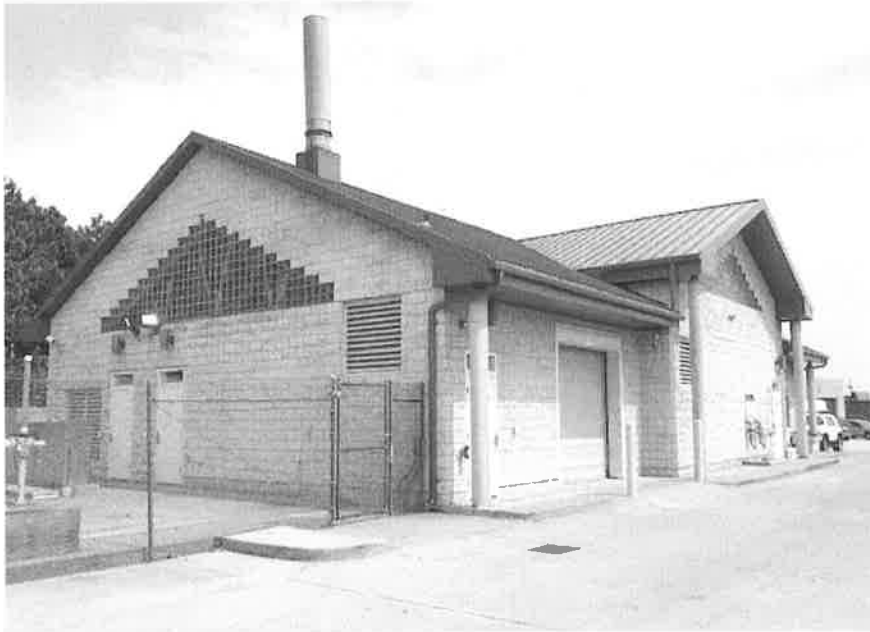
(L) Water & Sewage Department Building - looking southeast
