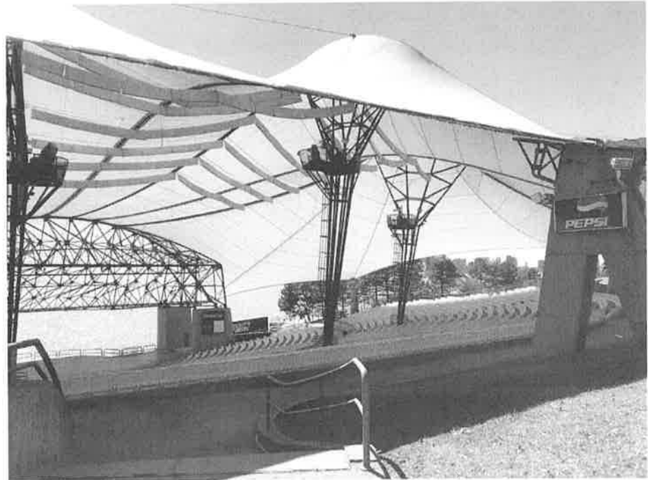
(I) Tensile Roof over Fixed Seating-Looking south
