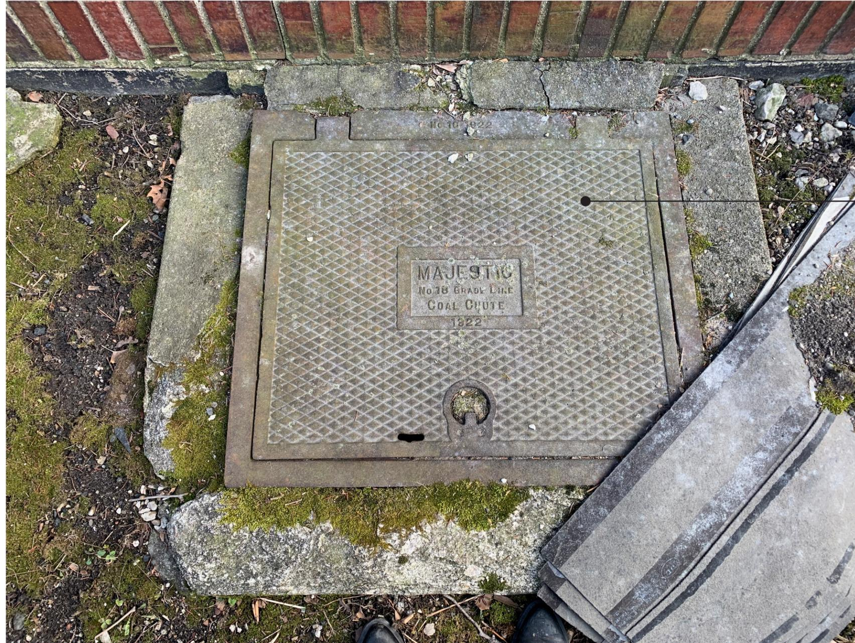
EXISTING COAL CHUTE DOOR TO BE REMOVED. ALL WALLS BELOW GRADE TO BE REMOVED. HOLE IN BASEMENT WALL TO BE CLOSED IN WITH CONCRETE. REMAINING HOLE TO BE FILLED WITH SOIL AND PREPPED FOR NEW DRIVEWAY
