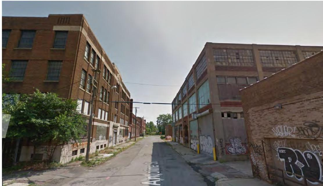
BUILDING 2/3 - CONCRETE FRAME WITH STEEL SASH GLAZING INFILL
