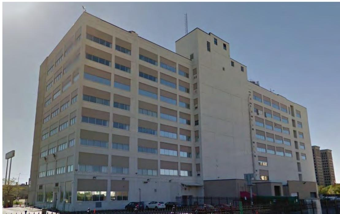
BUILDING 10 - CONCRETE FRAMED OPENINGS WITH STOREFRONT AND SPANDREL
