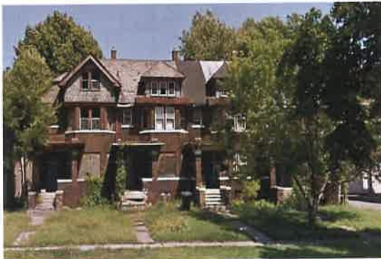
Property Before Renovation
