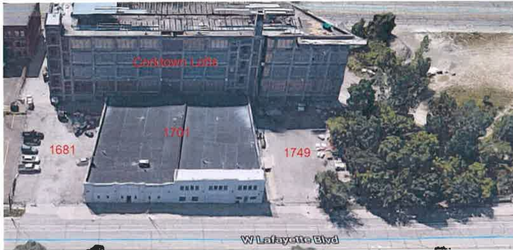
Figure 5. Previous Site Conditions: Adjoining Parking Structure (1701 W Lafayette)
